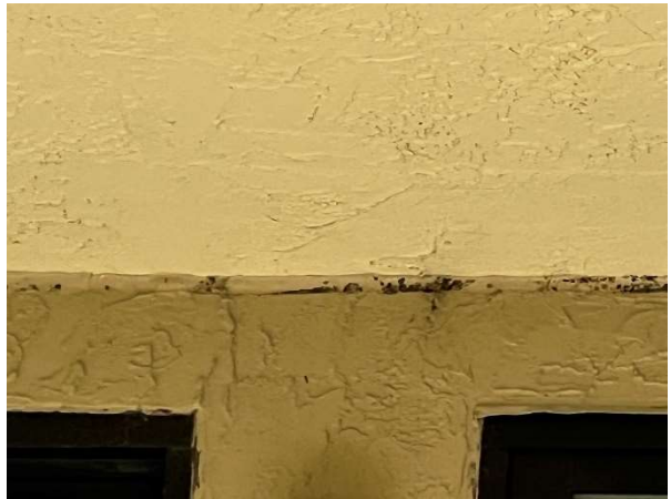
Deterioration at edge
