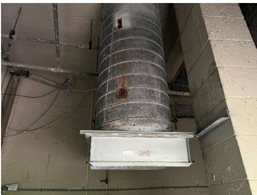
Minor rust formation at trash chute
