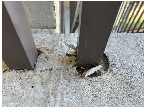
Spalled embedded connections
