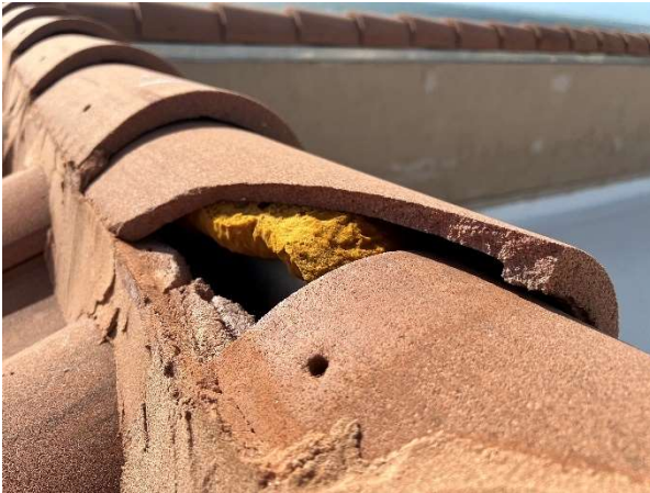
Damaged tile at rooftop
