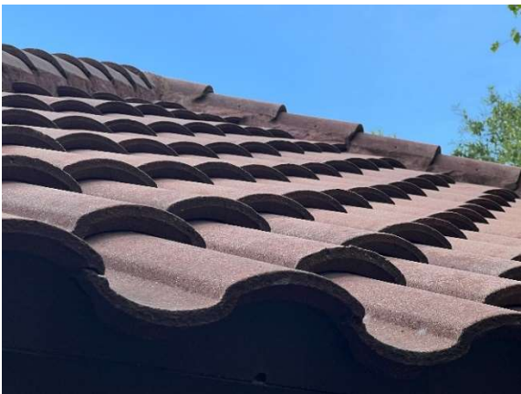
Concrete tile detail view
