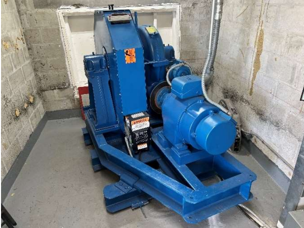
Elevator hoist and motor
