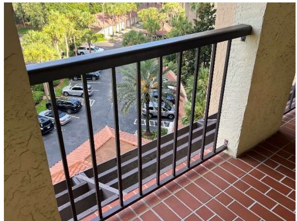
Railings mechanically attached
