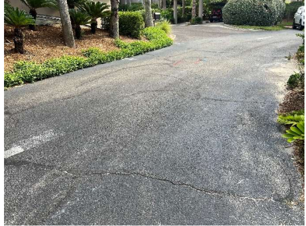
Cracks and previous repairs evident
