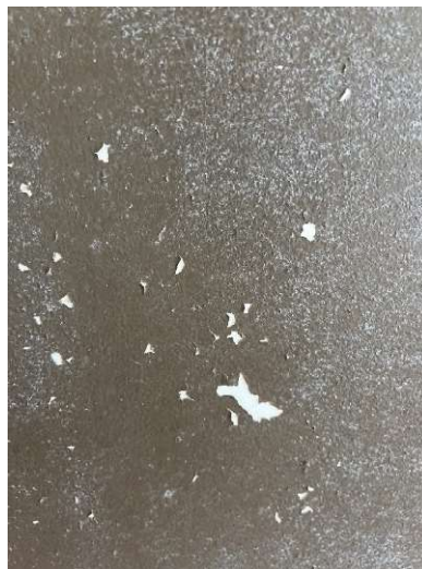
Finish deterioration
