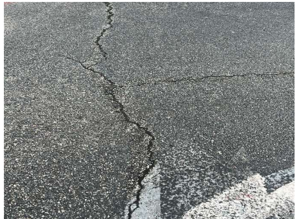
Cracks evident
