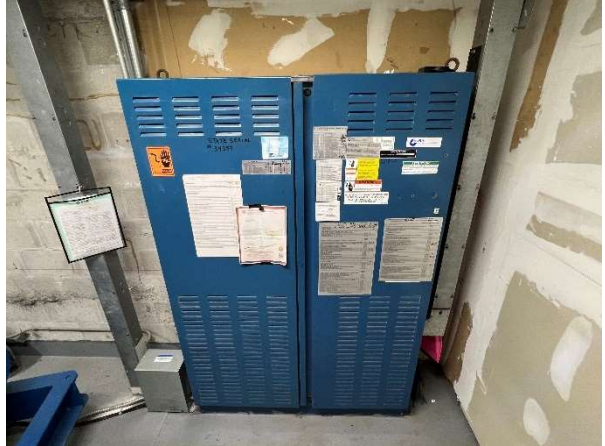
Elevator control cabinets
