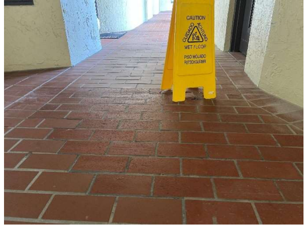
Area of buckled paver tiles
