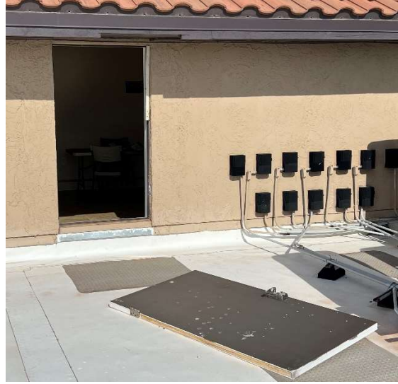
Hinge failure at rooftop door
