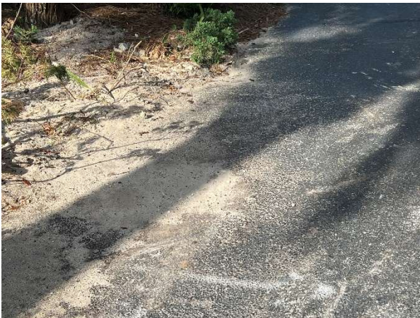
Sediment accumulation evident
