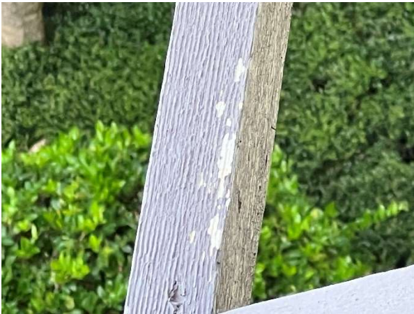
Finish deterioration
