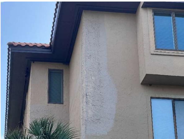
Stucco deterioration with previous repairs evident
