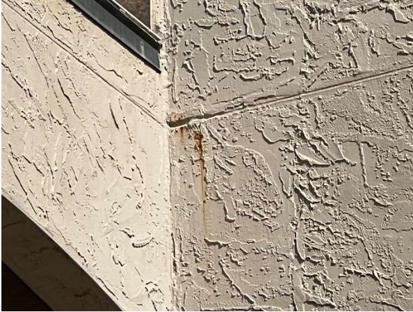
Rust stains near joint
