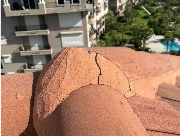
Minor mortar cracks
