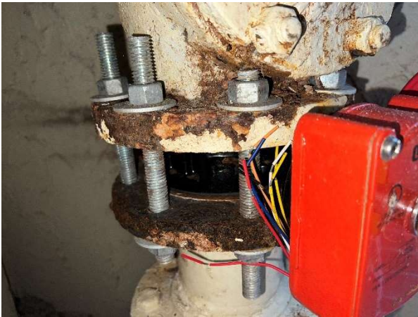
Rust evident at fire standpipe
