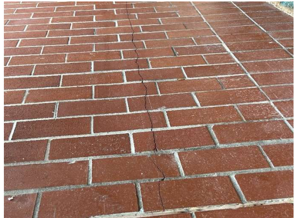
Cracked breezeway paver tiles
