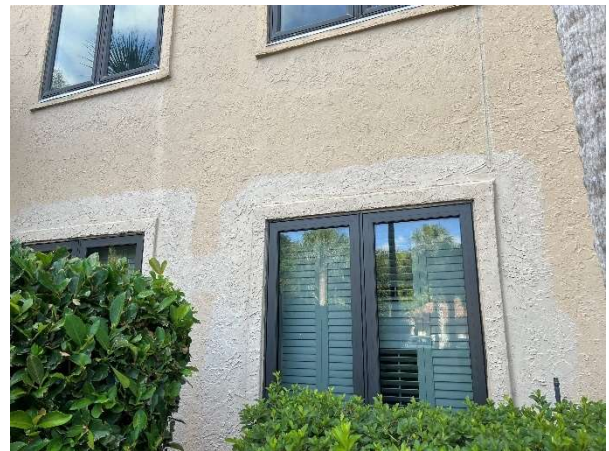
Previous repairs evident (inconsistent finishes)
