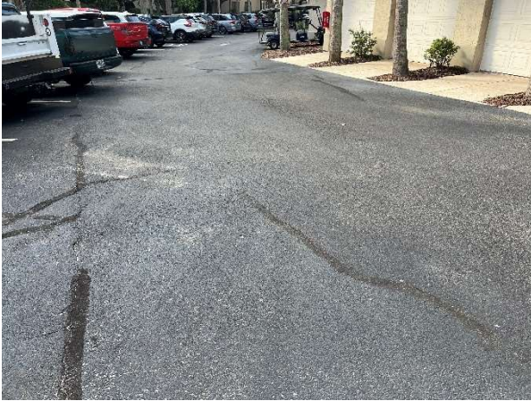
Cracks and previous repairs evident
