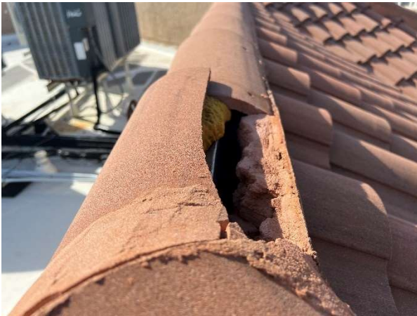
Damaged tile at rooftop
