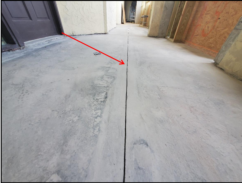
Photograph 16. 6 th floor completed hollow core seam repair with proper control joint.
