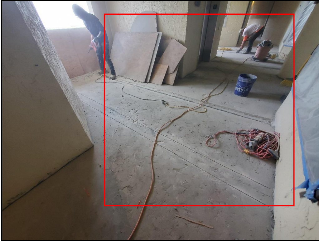
Photograph 14. 6 th floor hollow core seam repairs in progress.
