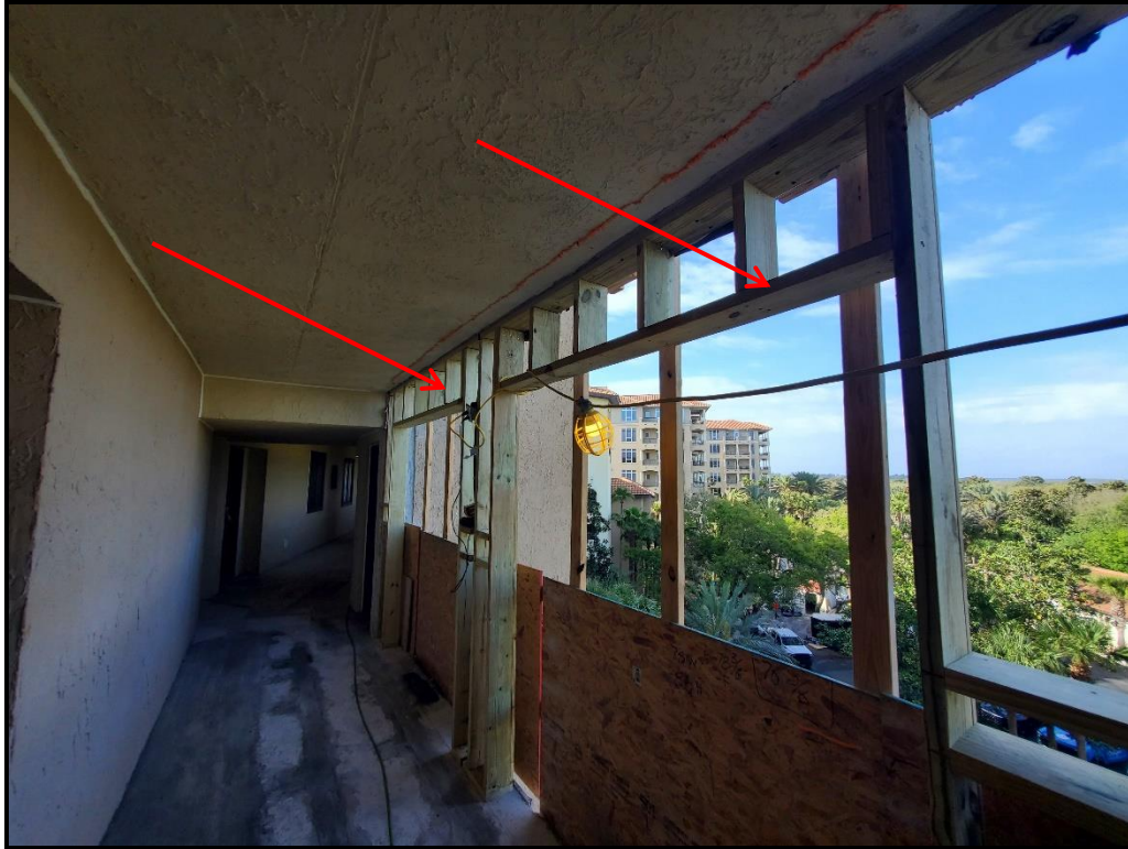
Photograph 6. 5 th floor archway framing installation in progress.
