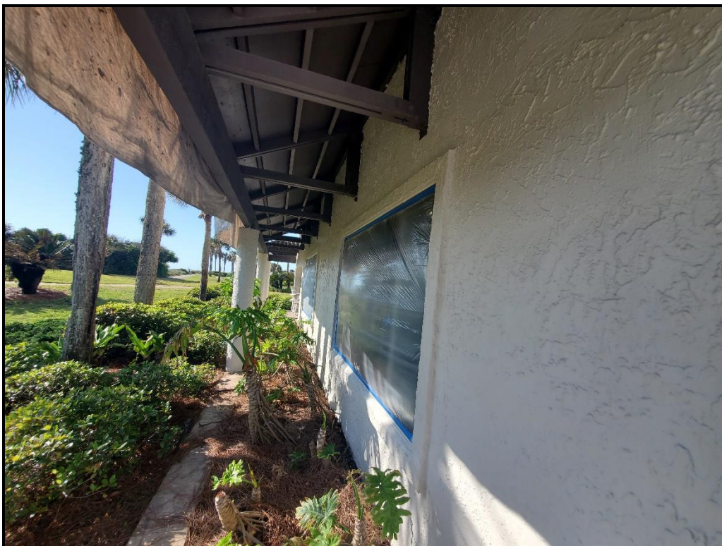
Photograph 19. Drop 3 wall coating application completed, punch in progress.
