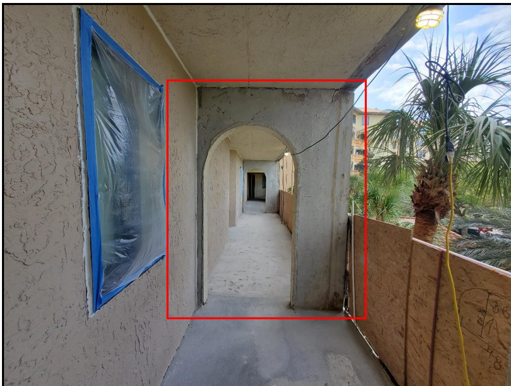
Photograph 7. Delaminated stucco repairs in progress.
