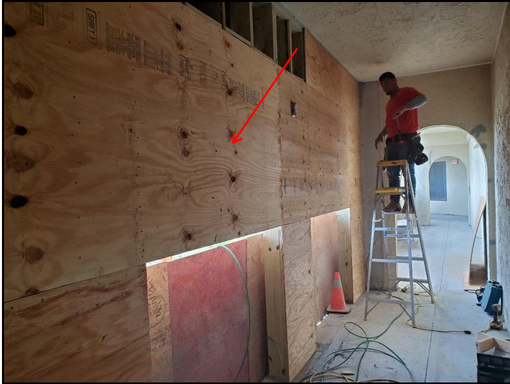
Photograph 12. 6 th floor archway sheathing installation in progress.
