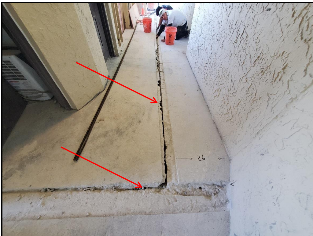
Photograph 3. 6 th floor hollow core panel seam repairs in progress.
