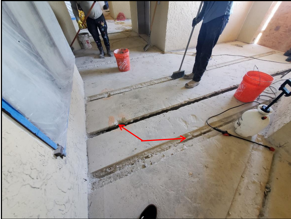
Photograph 4. 6 th floor hollow core panel seam repairs in progress.
