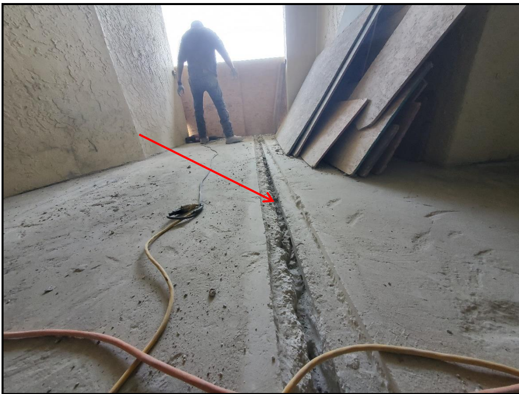
Photograph 15. 6 th floor hollow core seam repairs in progress.
