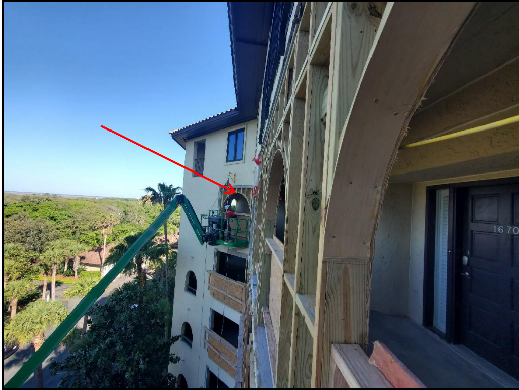
Photograph 22. 6 th floor archway sheathing installation in progress.
