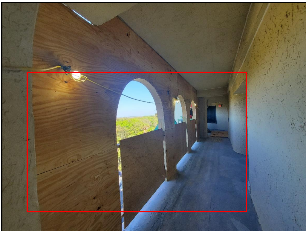
Photograph 21. 6 th floor archway sheathing installation in progress.
