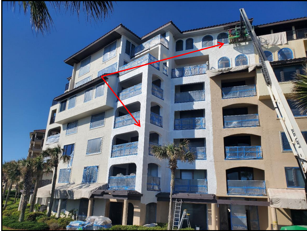
Photograph 20. Drop 3 topcoat nearing completion, Drop 4 primer coat application underway.
