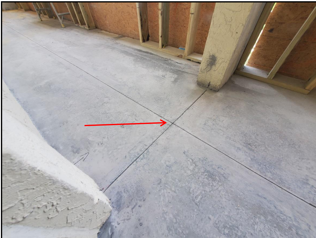
Photograph 17. 6 th floor completed hollow core seam repair with proper control joint.
