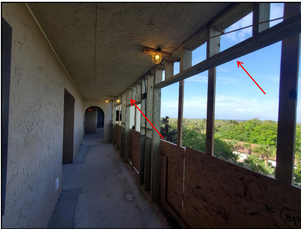
Photograph 5. 5 th floor archway framing installation in progress.
