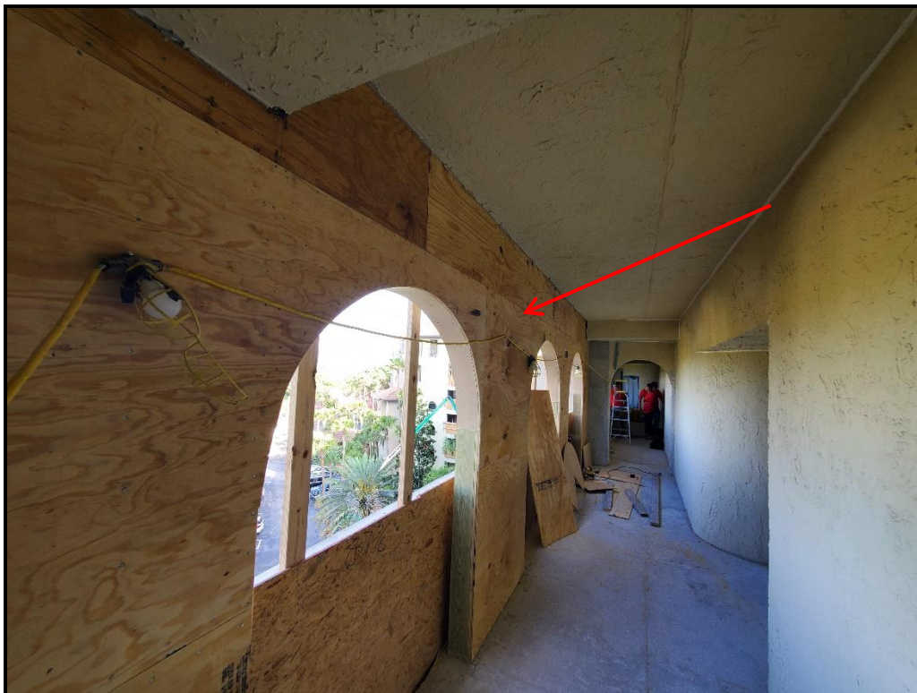
Photograph 1. 6 th floor archway sheathing installation in progress.
