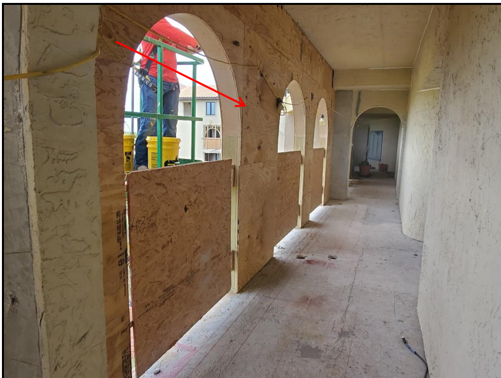
Photograph 11. 6 th floor archway rebuilds in progress.
