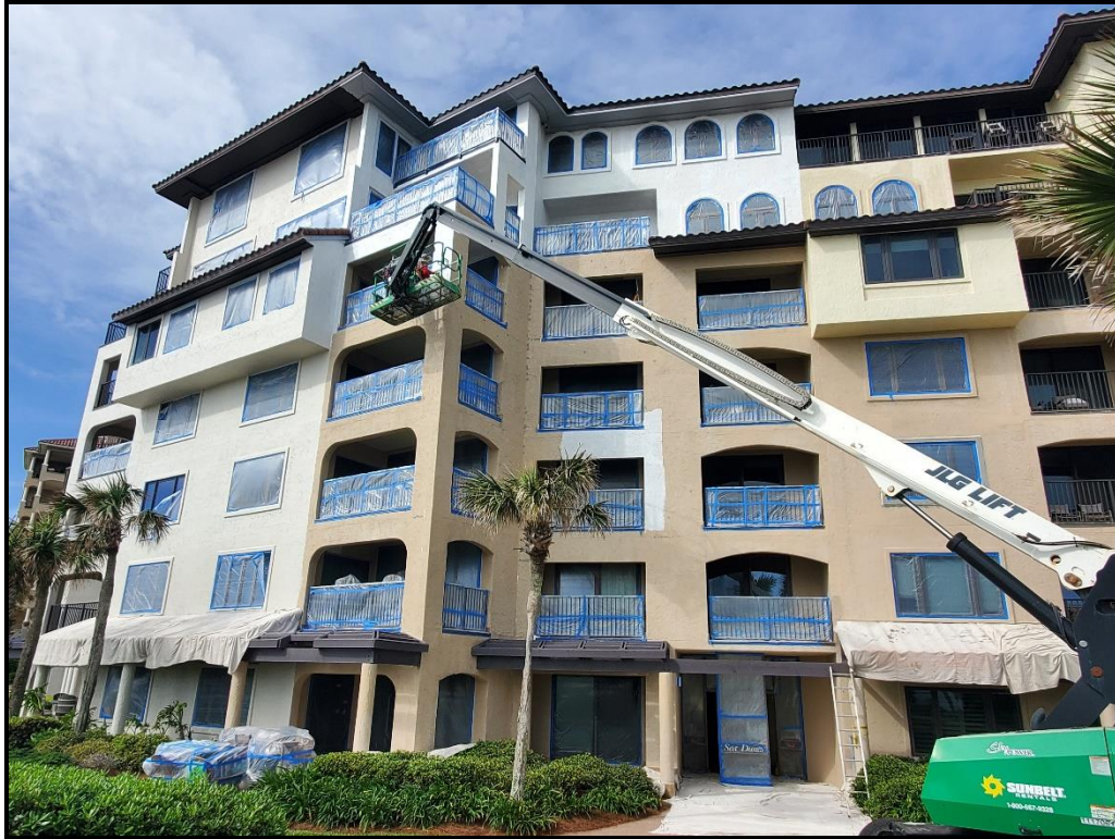
Photograph 10. Drop 3 & 4 protection re-installed and primer coat application in progress.
