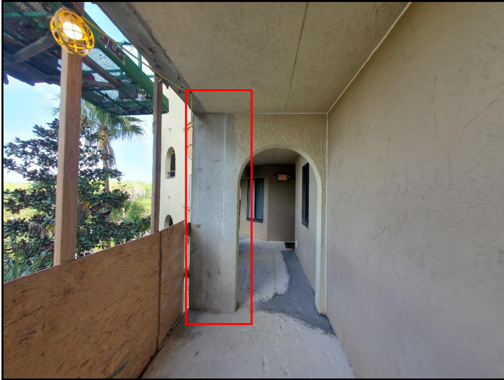
Photograph 8. Delaminated stucco repairs in progress.
