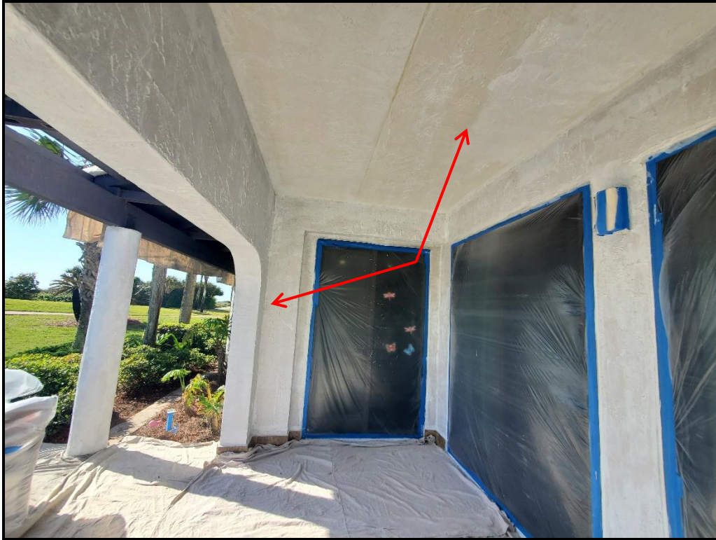
Photograph 18. Drop 4 primer coat application in progress.
