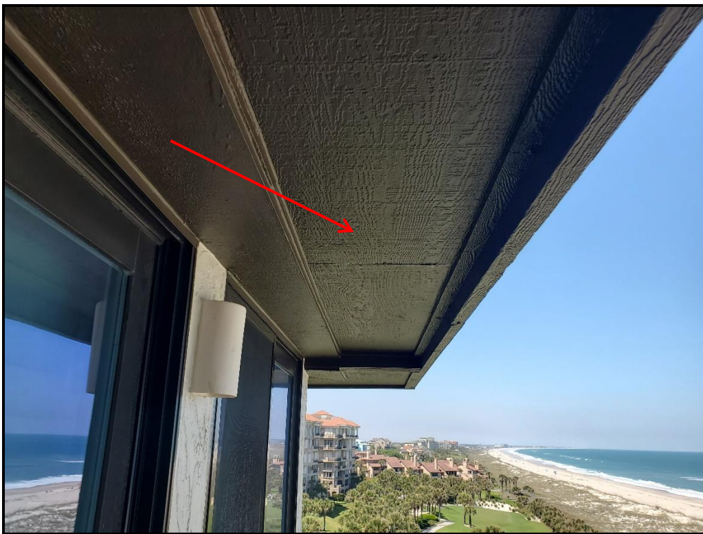
Photograph 3. Drop 3 soffit coating application complete.
