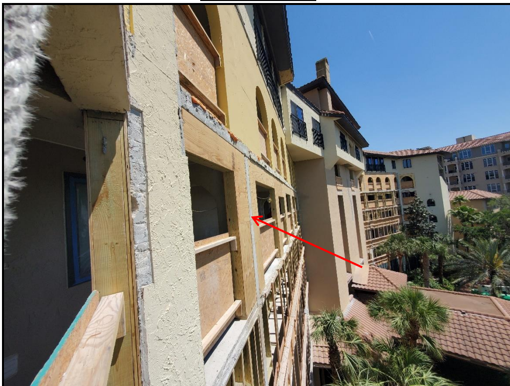
Photograph 11. 5 th floor archway rebuilds in progress.
