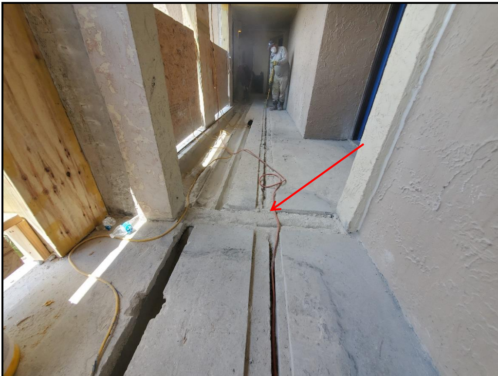
Photograph 13. 5 th floor hollow core seam repairs in progress.
