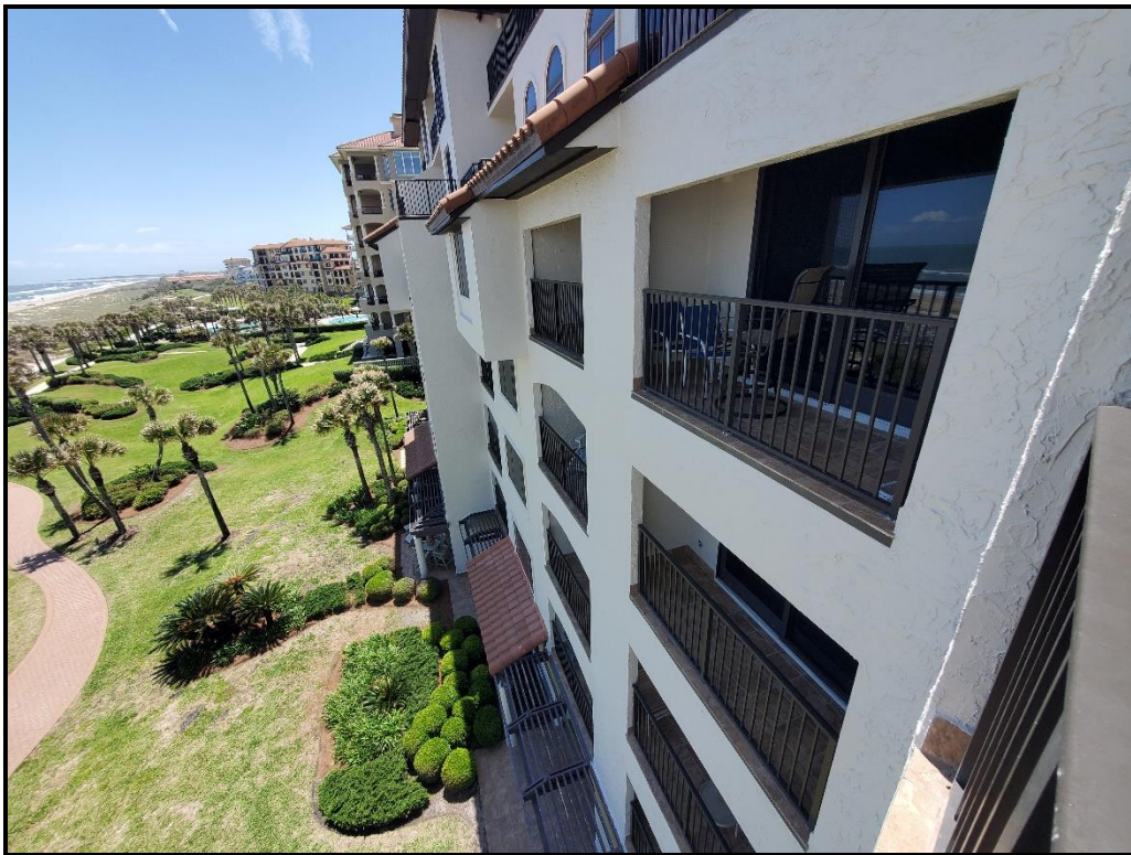
Photograph 21. Drop 3 coating application complete.
