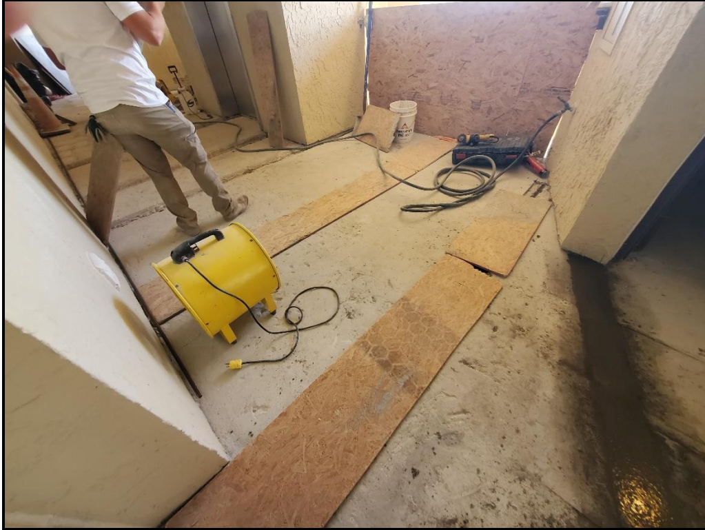
Photograph 8. 5 th floor hollow core seam repairs in progress.
