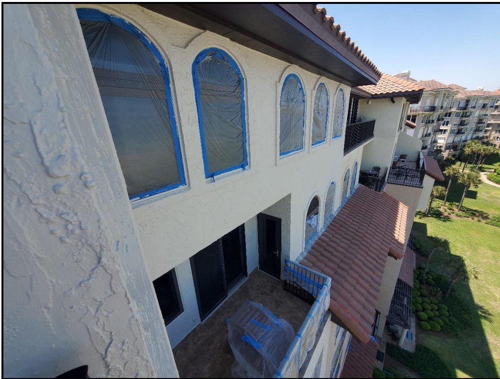
Photograph 5. Drop 3 wall coating application complete.
