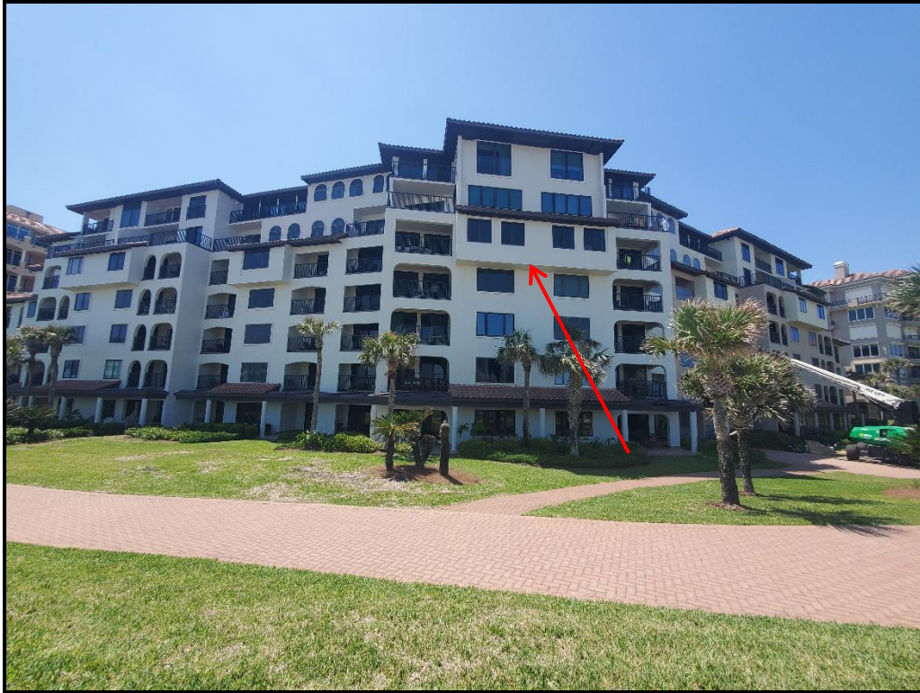
Photograph 2. Drop 3 coating application complete, punch work in progress.
