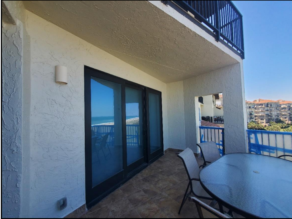
Photograph 4. Drop 3 wall coating application complete.
