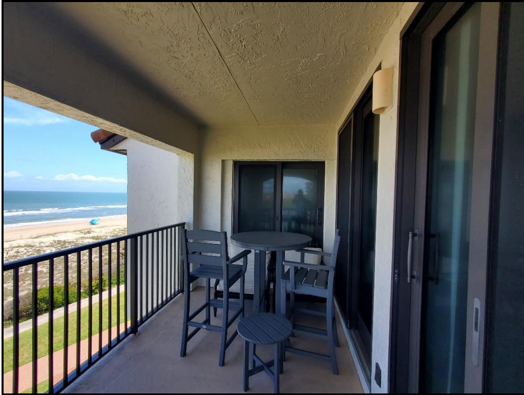
Photograph 22. Drop 3 coating application complete.
