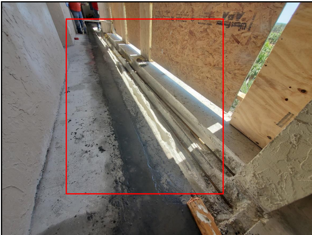
Photograph 7. 5 th floor hollow core seam repairs in progress.
