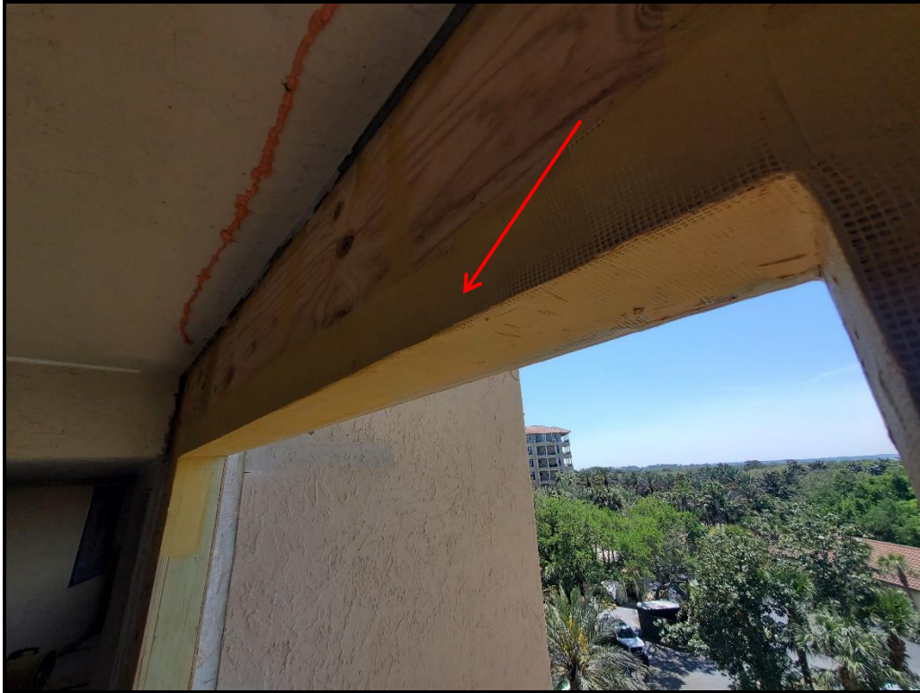
Photograph 12. 5 th floor archway and fluid applied weather barrier installation in progress.
