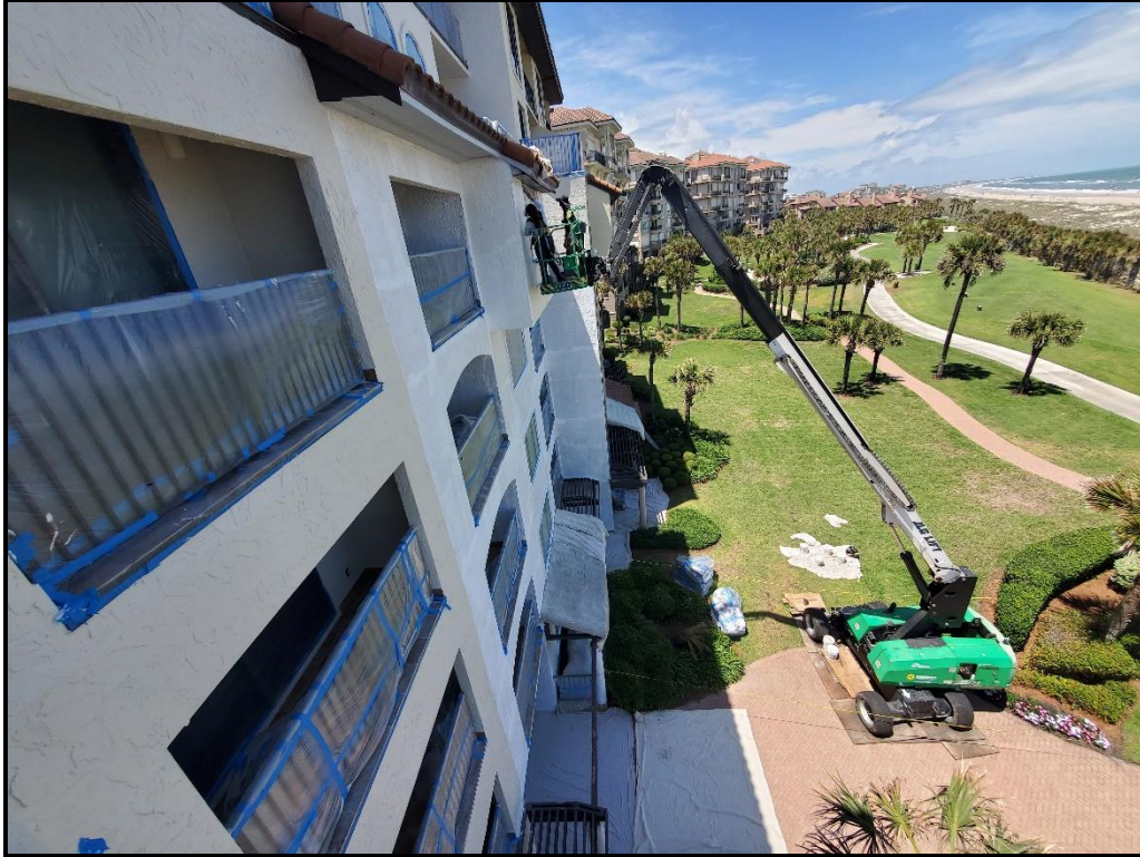
Photograph 24. Drop 4 topcoat application in progress.
