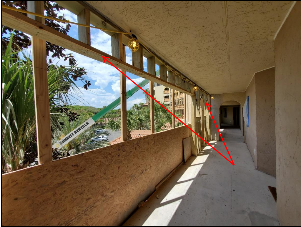
Photograph 18. 3 rd floor archway framing installation in progress.
