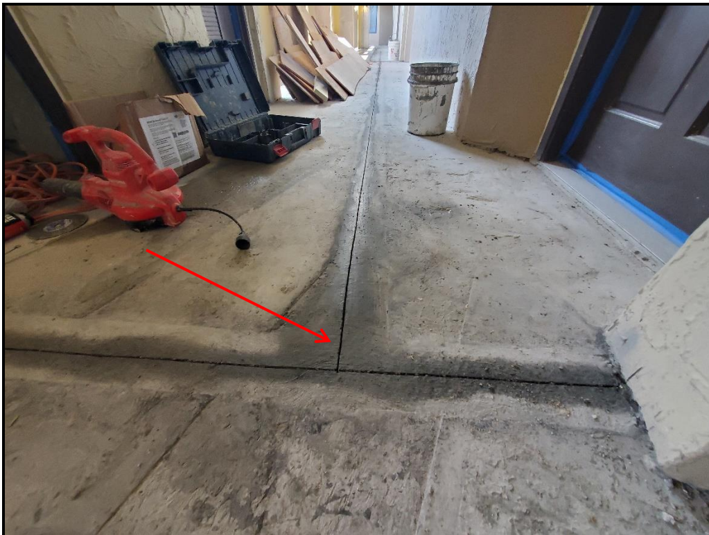
Photograph 15. 5 th floor hollow core seam repairs in progress.
