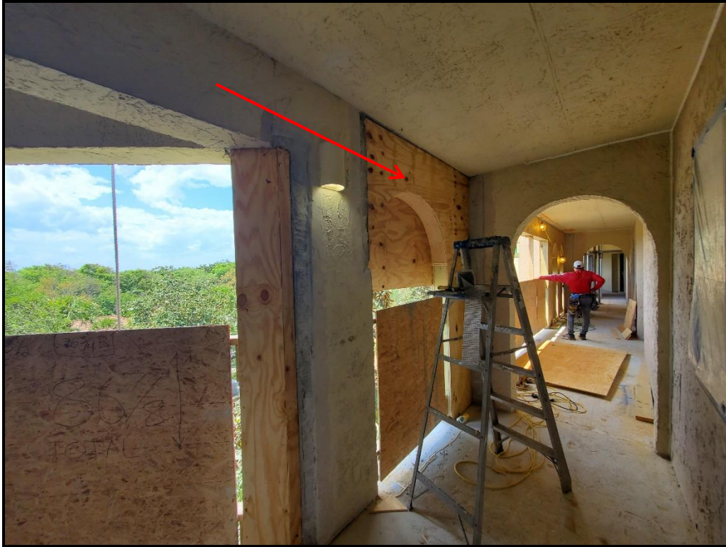
Photograph 16. 4 th floor archway sheathing installation in progress.
