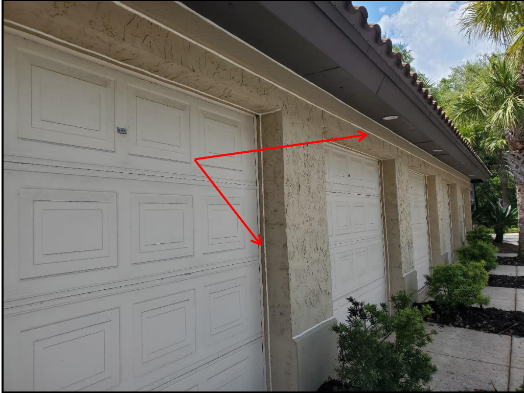
Photograph 20. Staloned garage sealant application nearing completion.
