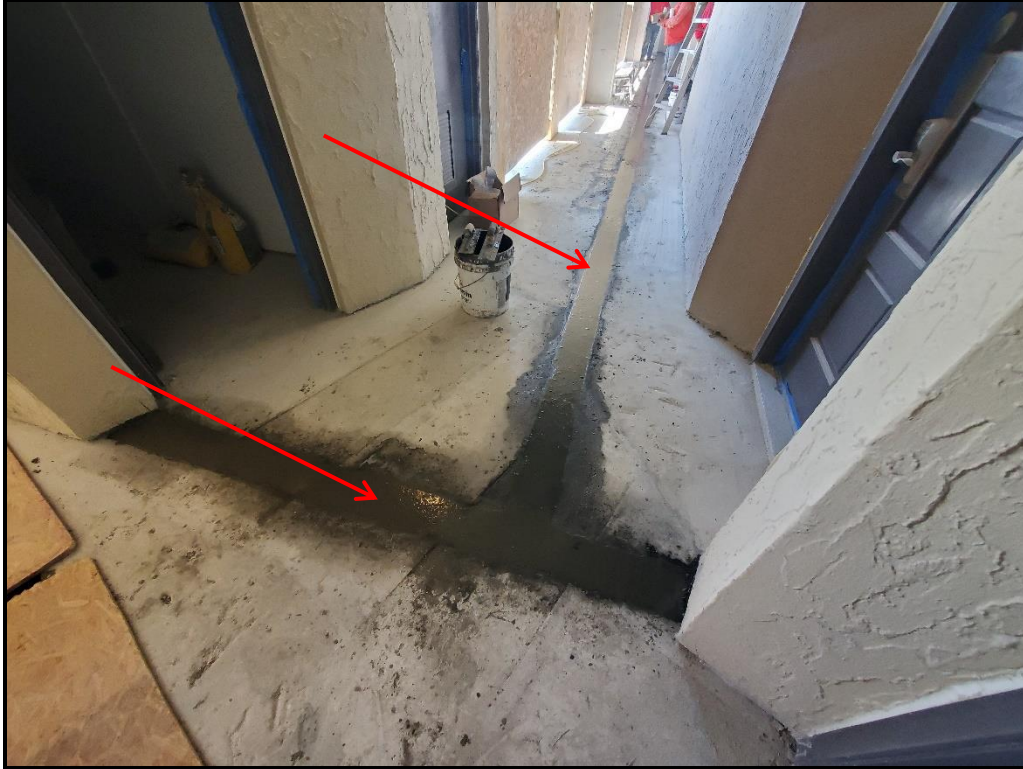
Photograph 6. 5 th floor hollow core seam repairs in progress.
