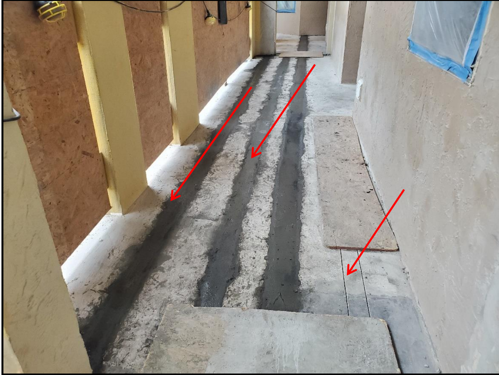
Photograph 12. 3 rd floor hollow core seam repairs in progress.
