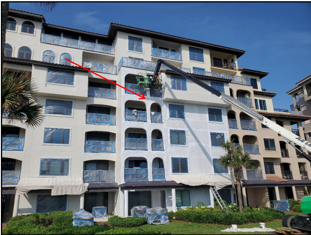
Photograph 5. Drop 4 primer coat application in progress.
