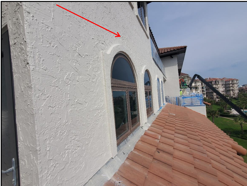
Photograph 3. Drop 3 wall coating application completed.
