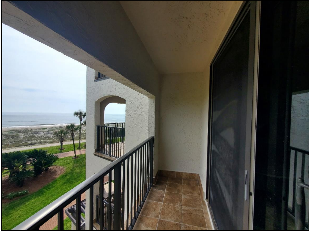
Photograph 4. Drop 3 wall coating application completed.
