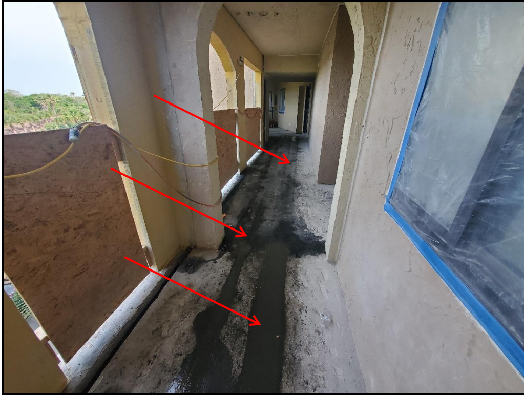
Photograph 8. 4 th floor hollow core seam repairs in progress.
