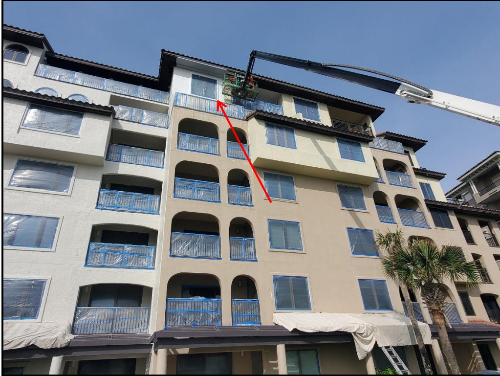
Photograph 2. Drop 4 primer coat application in progress.
