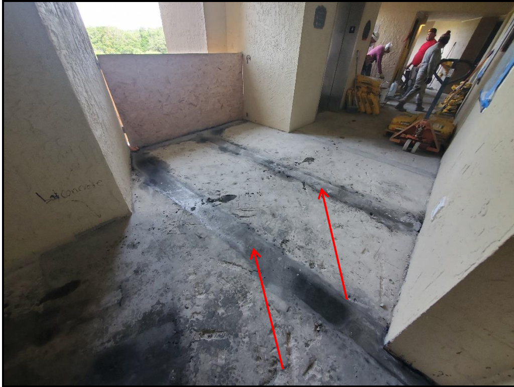
Photograph 10. 4 th floor hollow core seam repairs in progress.
