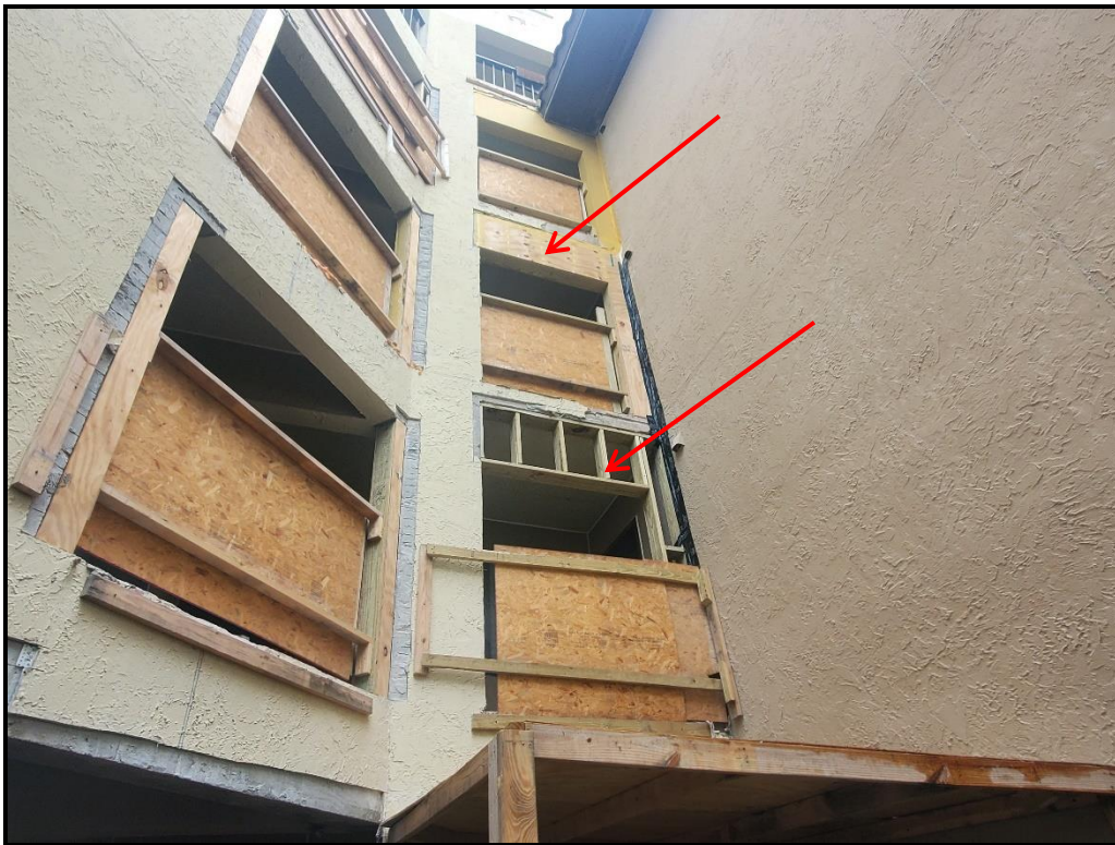
Photograph 13. Archway rebuilds nearing completion.
