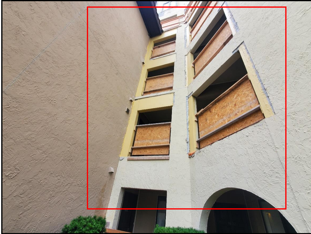
Photograph 14. Archway rebuilds nearing completion.
