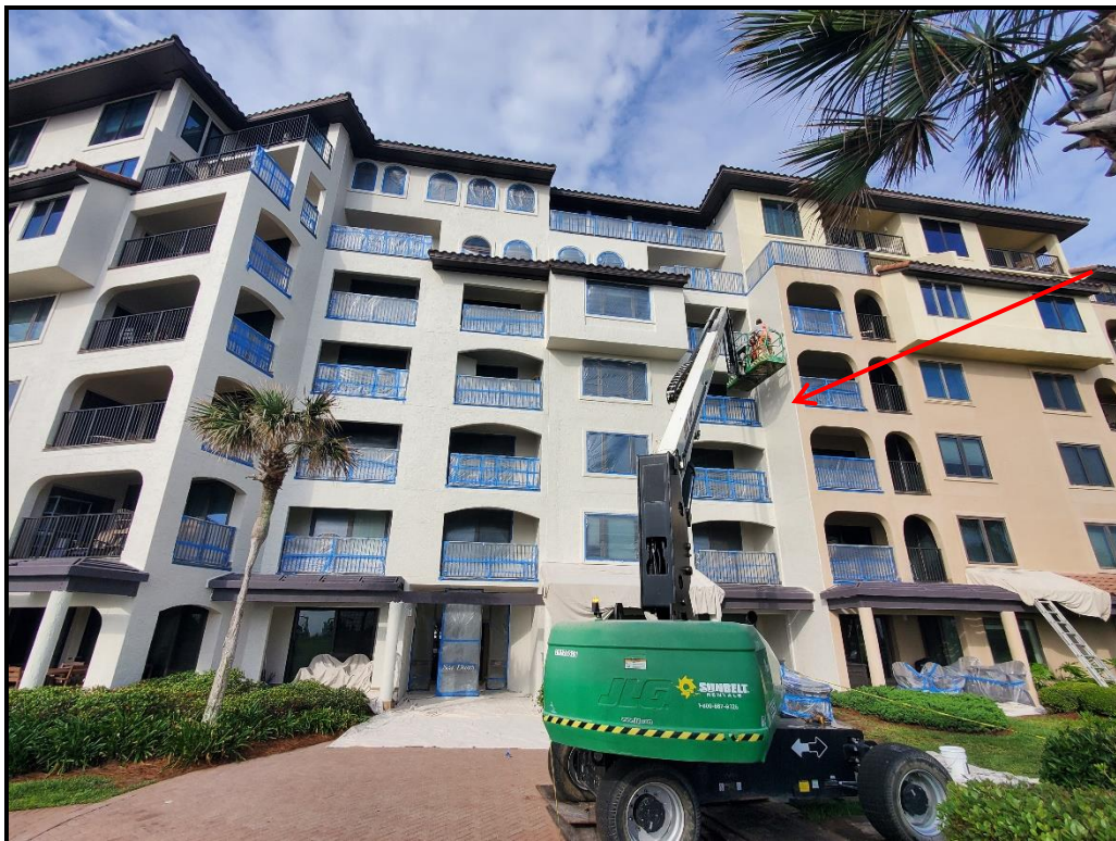
Photograph 1. Drop 4 top coat application in progress.
