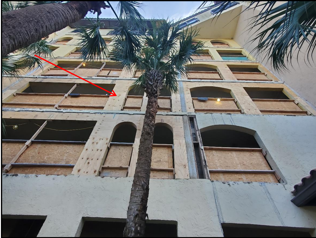
Photograph 6. Northwest elevation archway rebuilds nearing completion.
