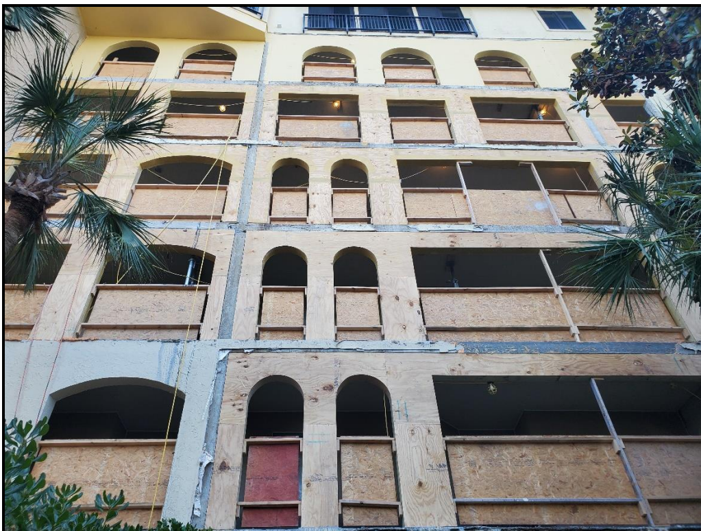
Photograph 7. Southwest elevation archway rebuilds nearing completion.
