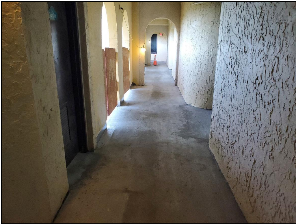
Photograph 7. 6 th floor walkway sloping completed.
