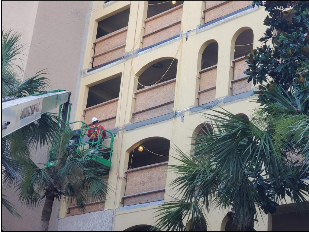
Photograph 12. West elevation stucco application and edge metal details in progress.
