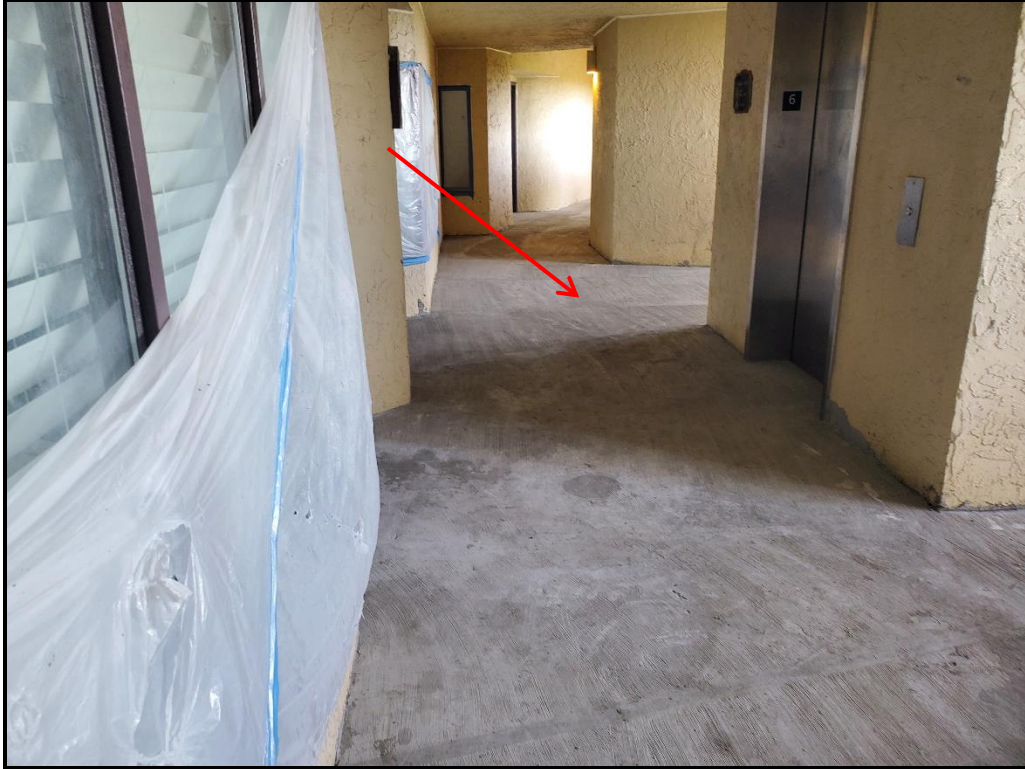
Photograph 6. 6 th floor walkway sloping completed.
