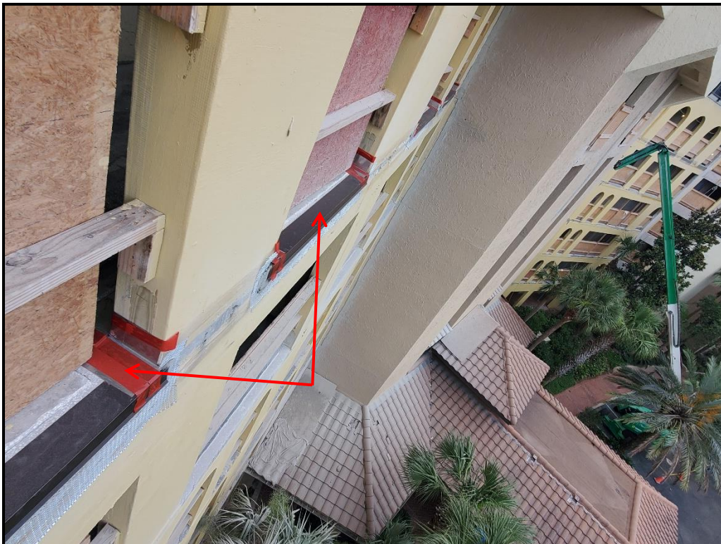
Photograph 5. 6 th floor west walkway flashing and drip edge installation in progress.
