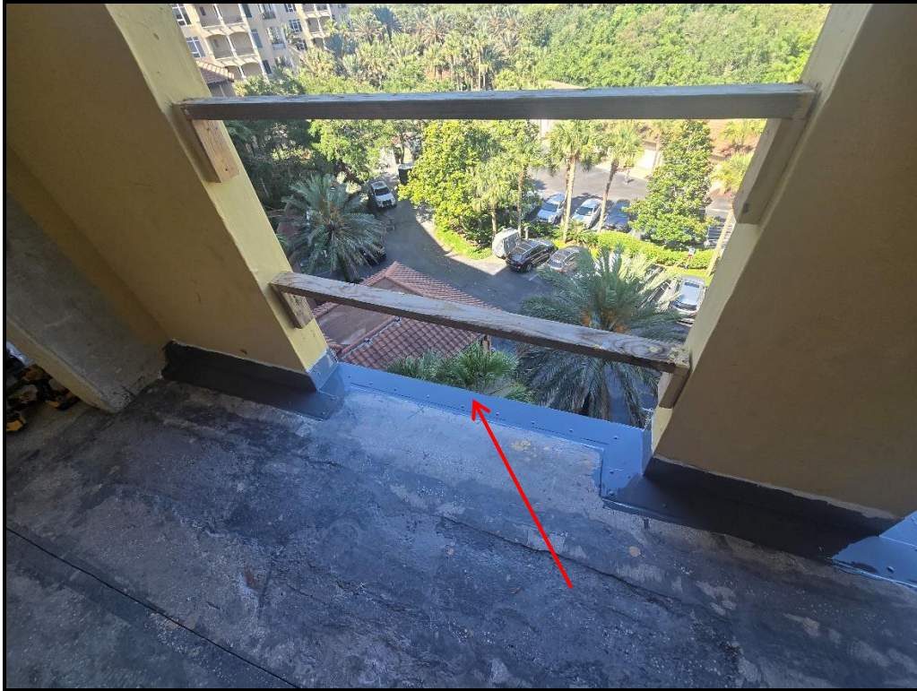
Photograph 2. 6 th floor west walkway flashing, drip edge and waterproofing detail installation in progress.
