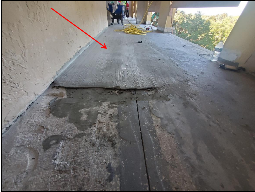
Photograph 10. 5 th floor sloping application in progress.
