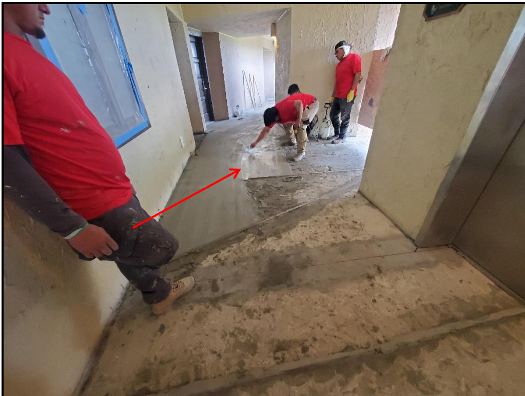
Photograph 11. 5 th floor sloping application in progress.
