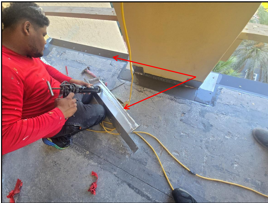
Photograph 1. 6 th floor west walkway flashing and drip edge installation in progress.
