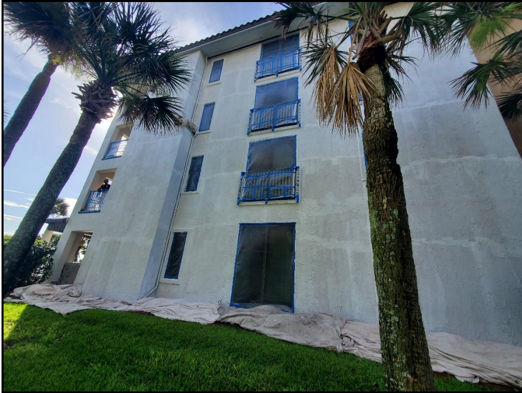
Photograph 8. North elevation primer coat application in progress.
