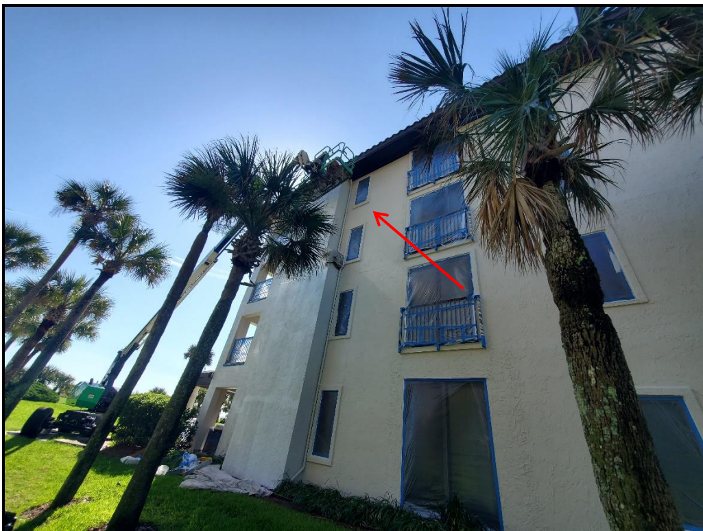
Photograph 9. North elevation topcoat application in progress.
