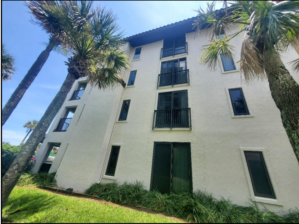
Photograph 14. North elevation wall coating completed.
