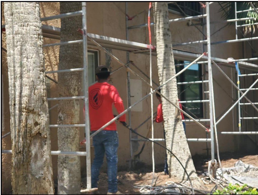
Photograph 15. South elevation pressure washing in progress.
