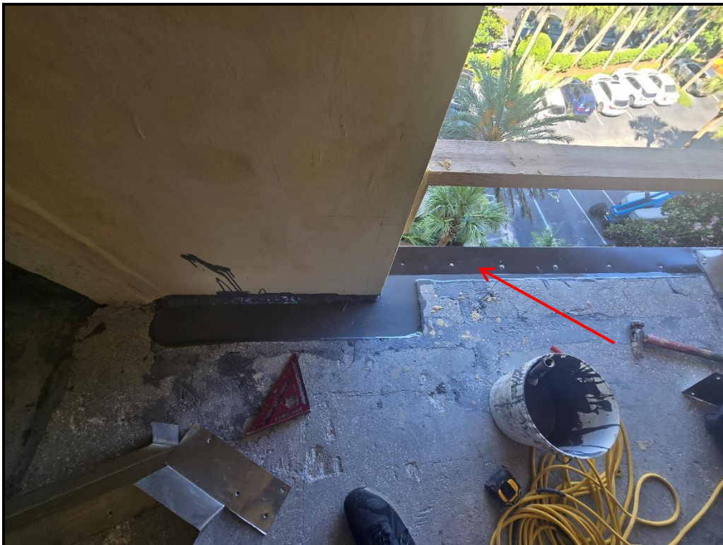
Photograph 3. 6 th floor west walkway flashing, drip edge and waterproofing detail installation in progress.
