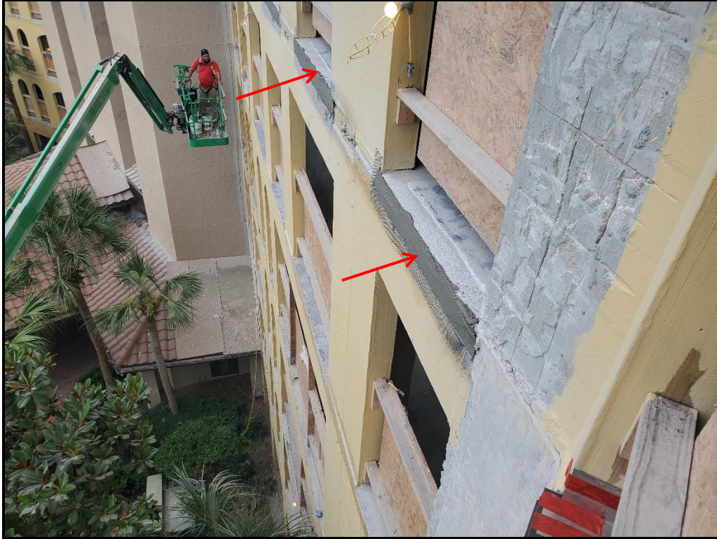
Photograph 4. West elevation stucco installation at slab edge in progress.
