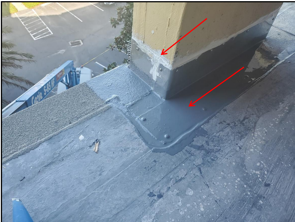
Photograph 13. 5 th floor flashing and edge metal waterproofing details in progress.
