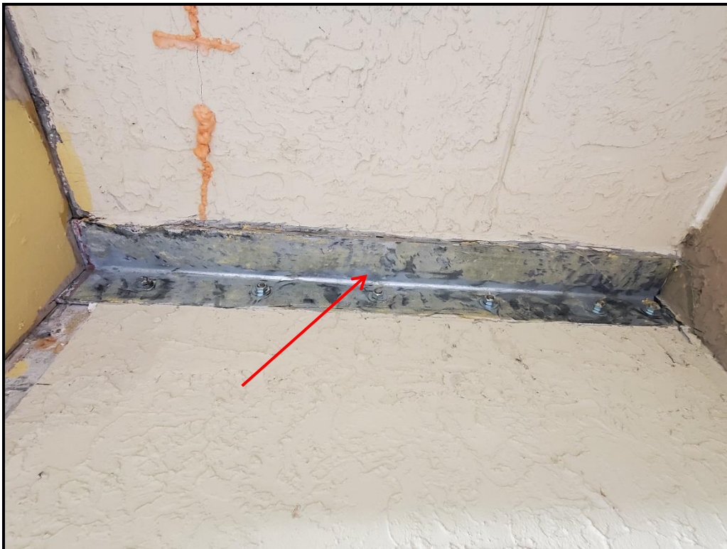
Photograph 11. 3 rd floor hollow core angle support corrosion treatment in progress.
