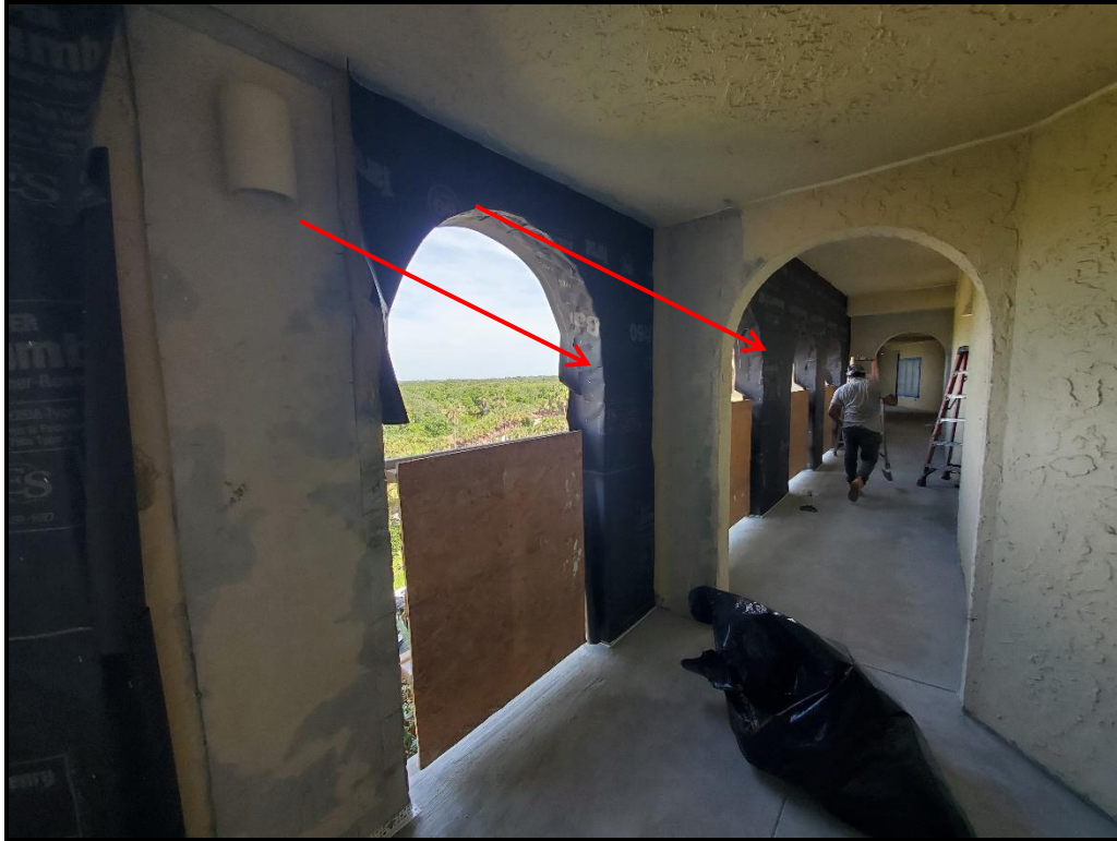
Photograph 14. 6 th floor west walkway stucco drainage paper installation in progress.
