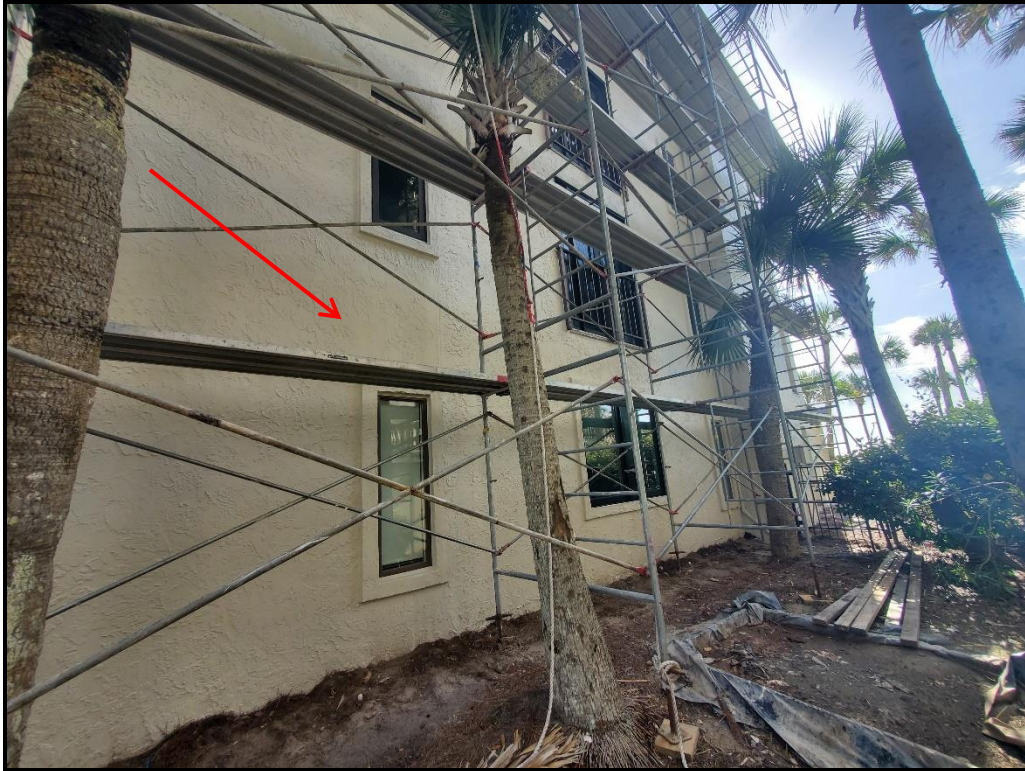
Photograph 6. South elevation wall coating application completed.
