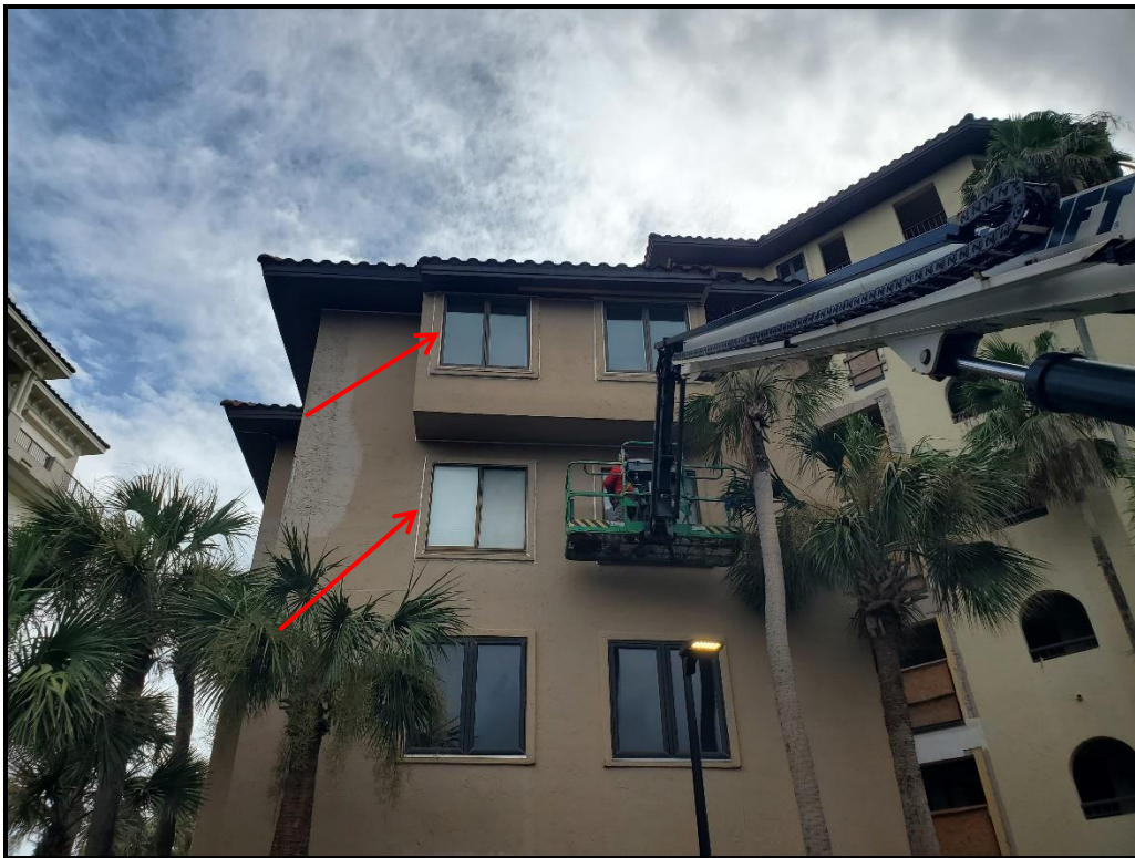
Photograph 5. West elevation new sealant application in progress on window stucco bands.
