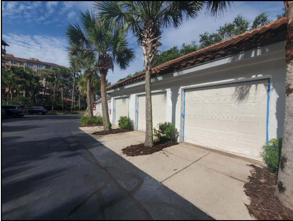
Photograph 8. Standalone garage primer coating application in progress.
