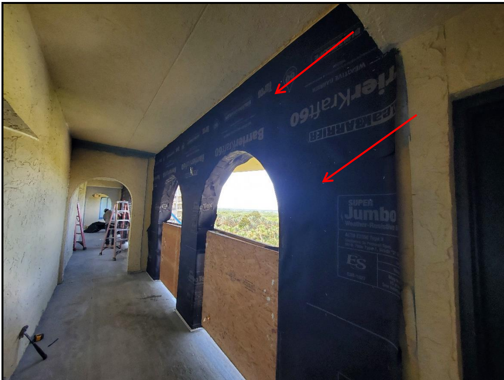
Photograph 13. 6 th floor west walkway stucco drainage paper installation in progress.
