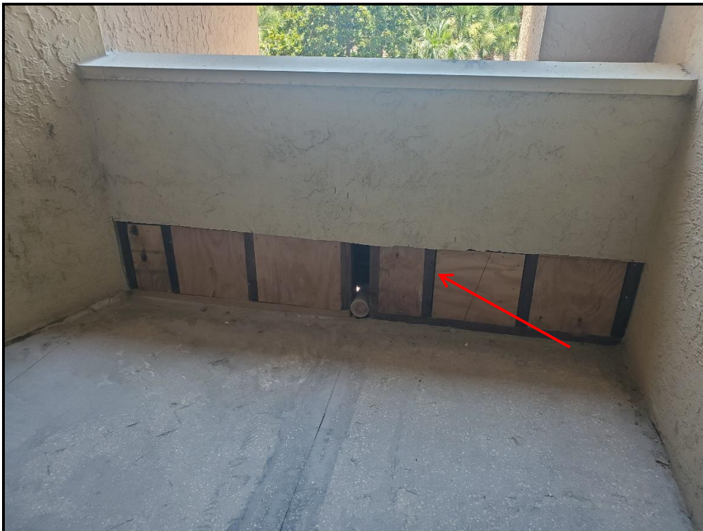
Photograph 3. 3rd floor west walkway knee wall repairs in progress
