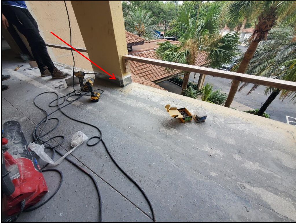
Photograph 10. 3 rd floor west walkway flashing, drip edge and waterproofing detail installation in progress.
