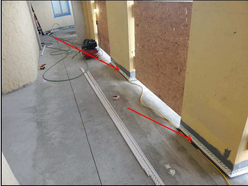
Photograph 12. 6 th floor archway stucco accessory installation in progress.
