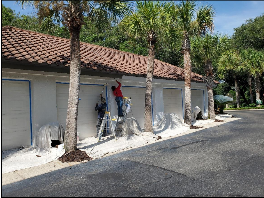
Photograph 16. Standalone garage top coat application in progress.
