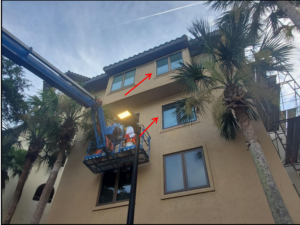
Photograph 4. West elevation new sealant application in progress on window stucco bands.
