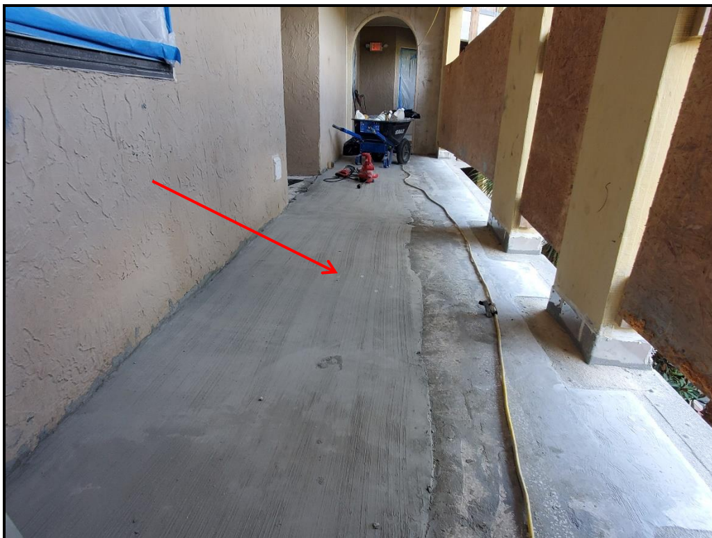
Photograph 15. 3 rd floor west walkway sloping application in progress.
