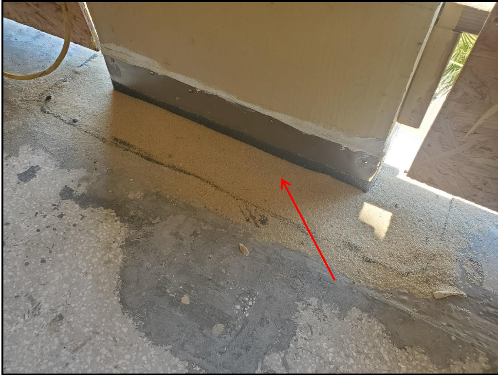
Photograph 2. 5 th floor west walkway flashing, drip edge and waterproofing detail installation in progress.
