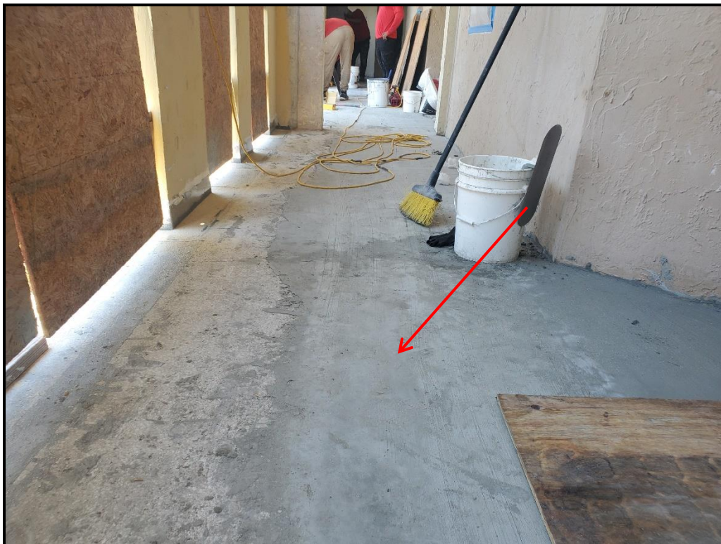
Photograph 1. 4 th floor west walkway sloping application in progress.
