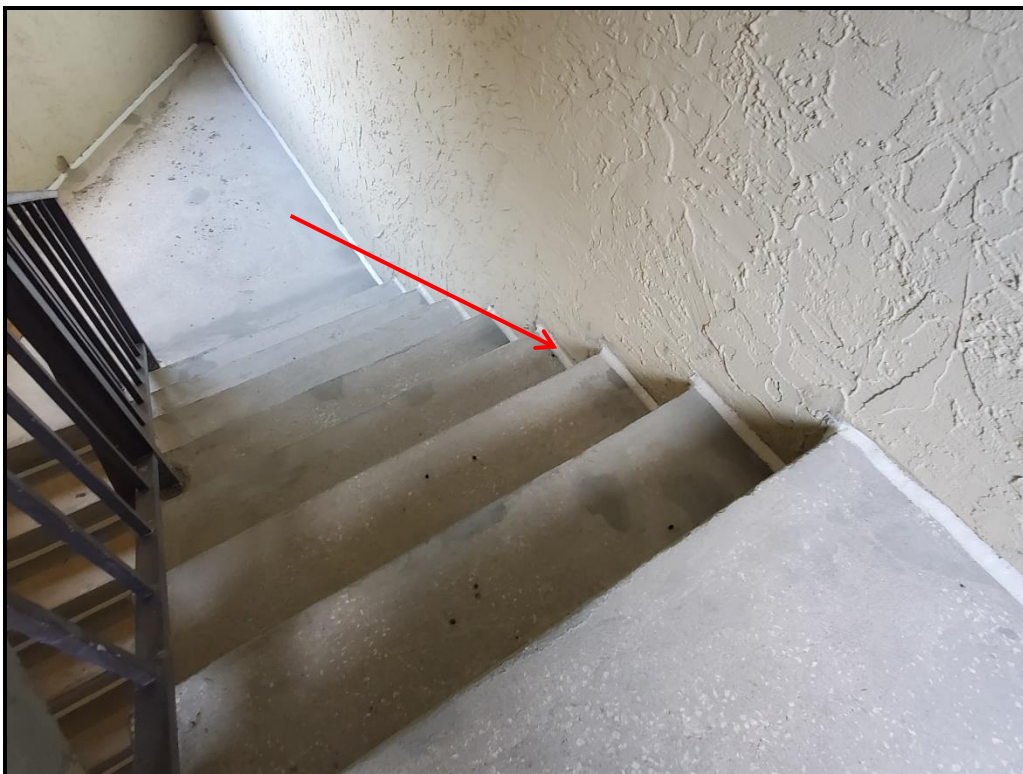
Photograph 15. South stair tower sealant application in progress.
