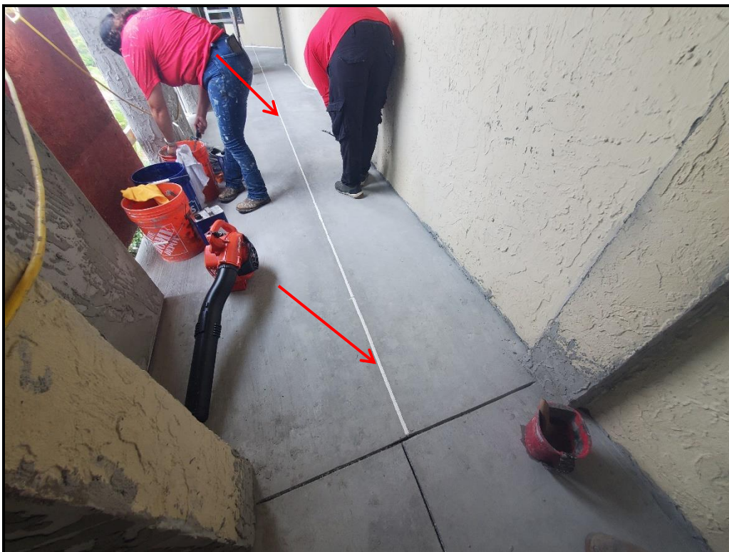
Photograph 17. 6 th floor sealant application in progress.
