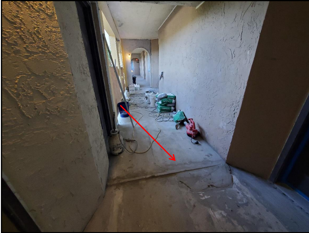
Photograph 8. 3 rd floor sloping installation in progress.
