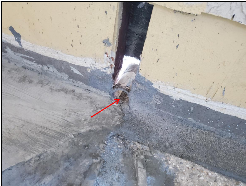
Photograph 5. Knee wall scupper drains modified & lowered to improve drainage.
