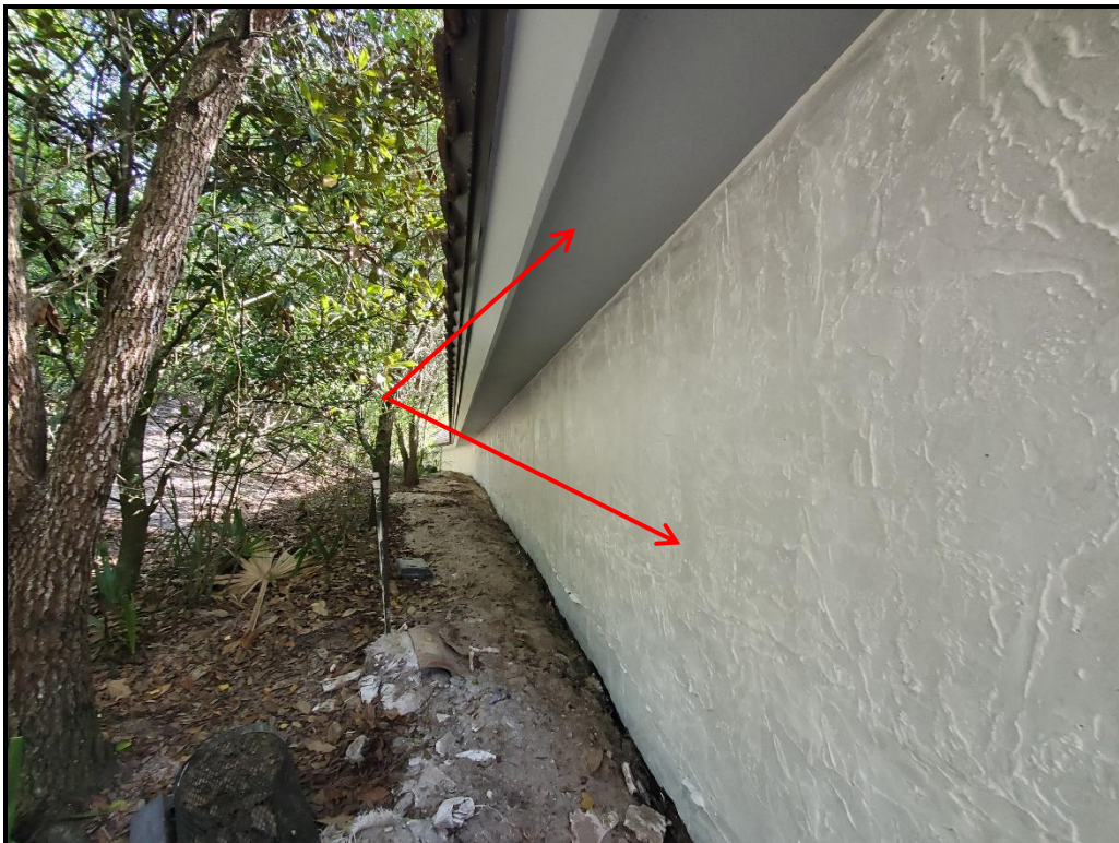
Photograph 11. Standalone garage wall and soffit primer coat application in progress.
