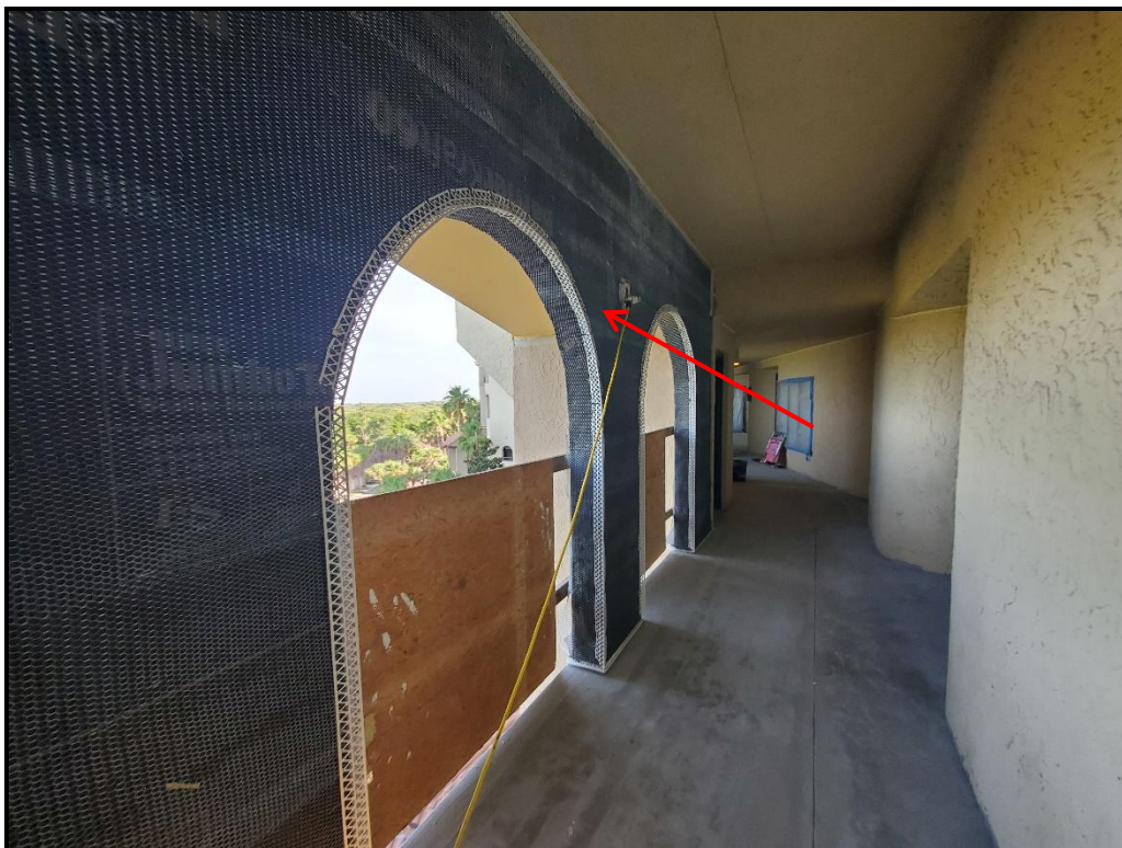
Photograph 3. 6 th floor west walkway stucco accessories and lath installation in progress.
