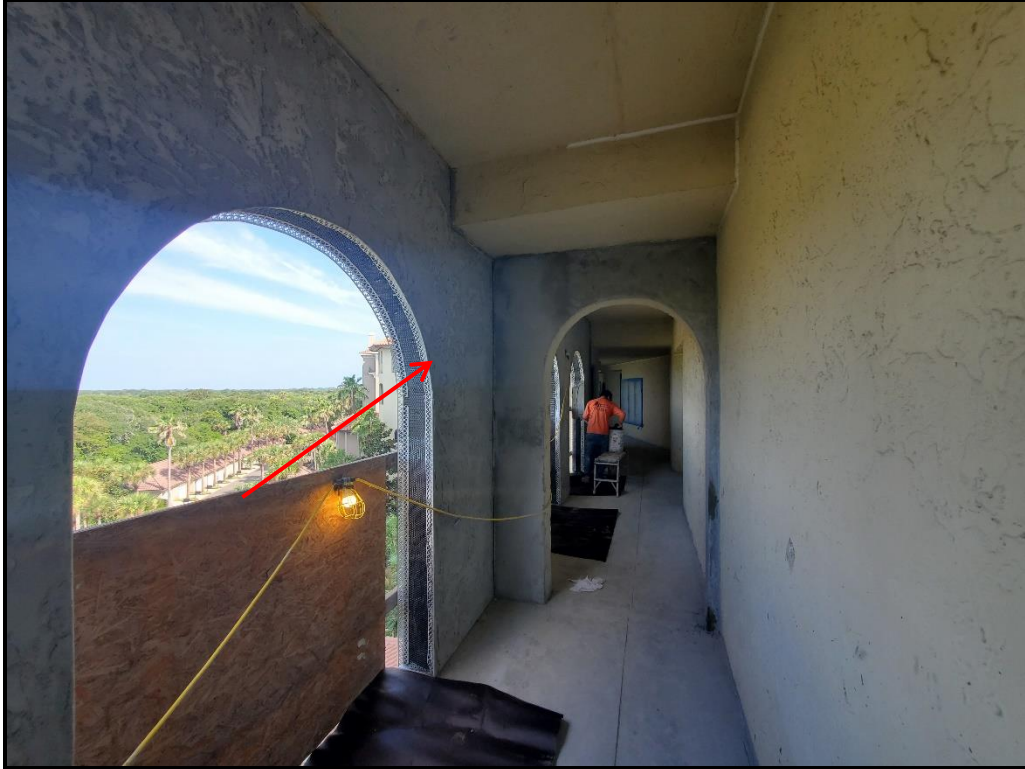
Photograph 12. 6 th floor archway stucco installation in progress.
