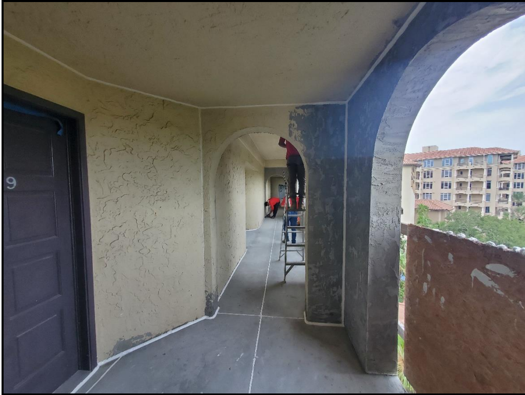
Photograph 16. 6 th floor sealant application in progress.
