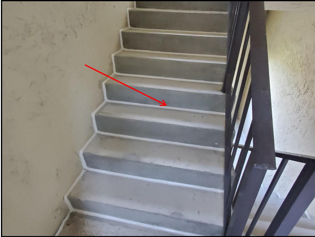
Photograph 14. South stair tower sealant application in progress.
