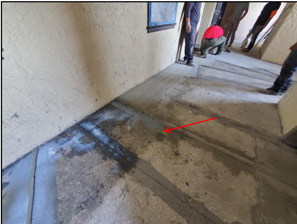
Photograph 9. 3 rd floor sloping installation in progress.
