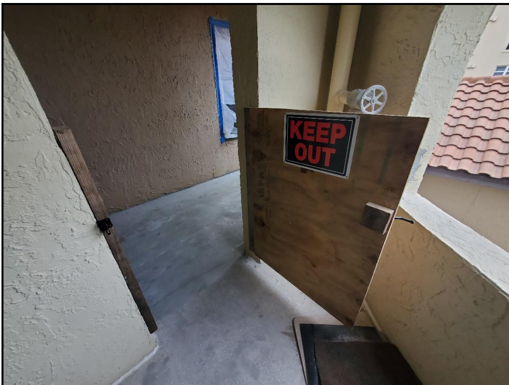
Photograph 19. South stair tower temporary gates installed.
