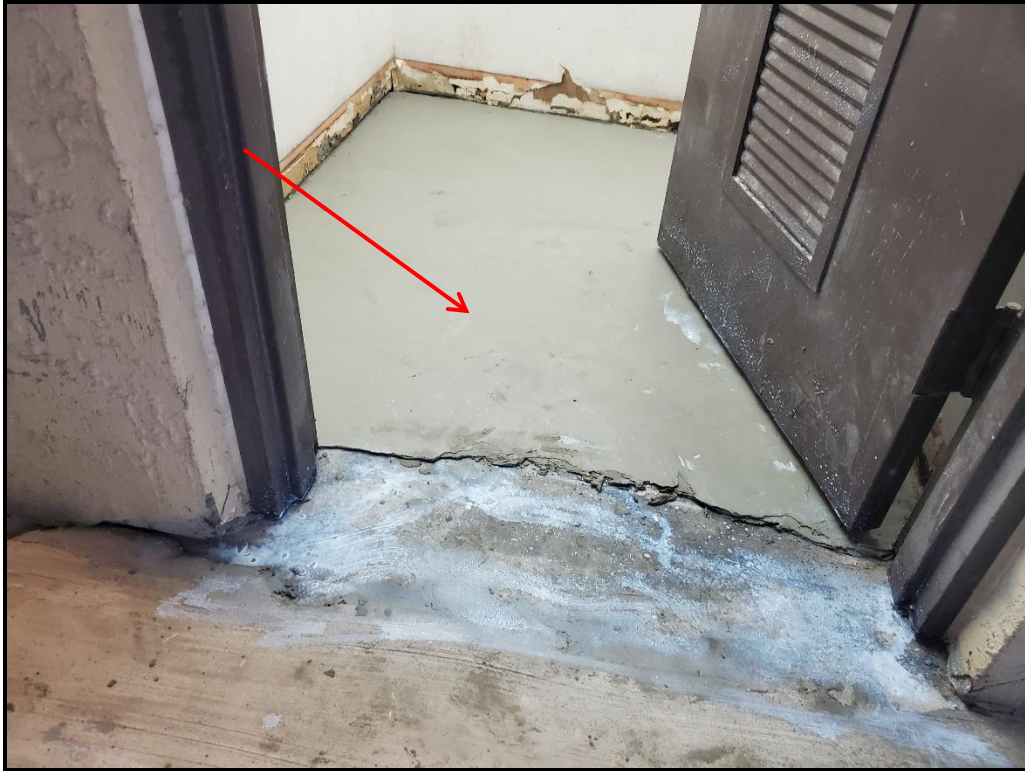
Photograph 10. Trash room floor sloping in progress.
