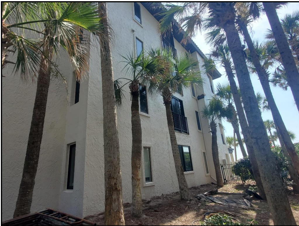
Photograph 7. South elevation wall coating application completed and scaffolding removed.
