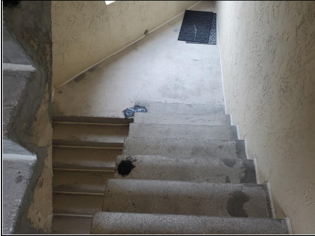
Photograph 20. South stair tower, handrails removed and concrete repairs in progress.
