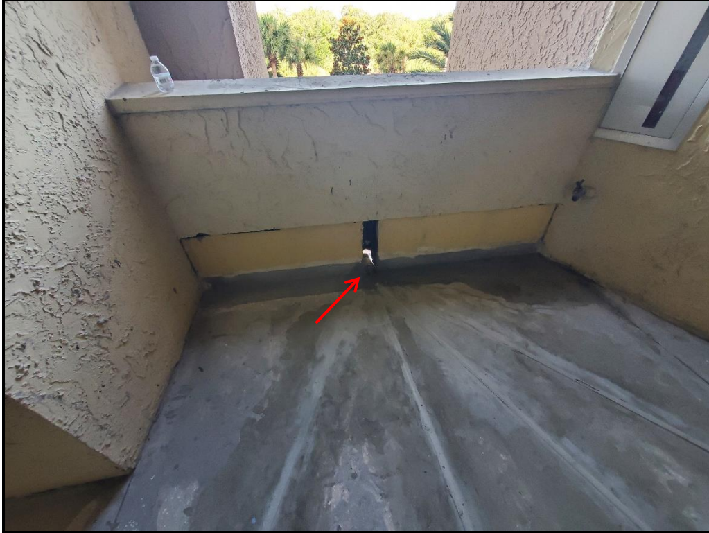
Photograph 4. Knee wall scupper drains modified & lowered to improve drainage.
