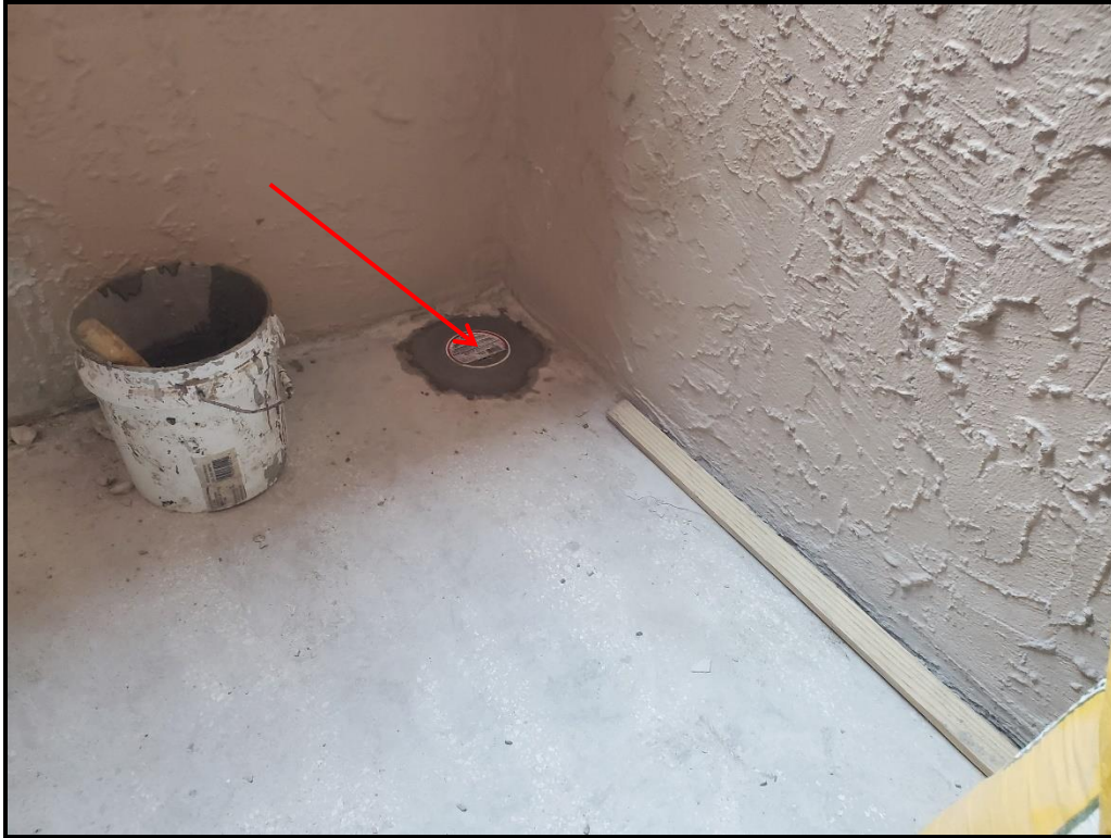
Photograph 6. Landing drains modified & lowered to improve drainage.
