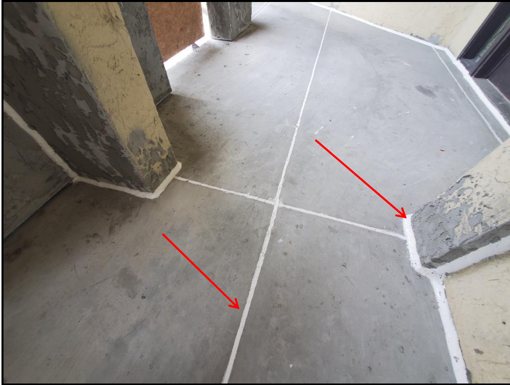
Photograph 18. 6 th floor sealant application in progress.
