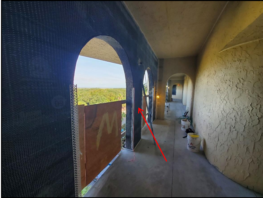
Photograph 2. 6 th floor west walkway stucco accessories and lath installation in progress.
