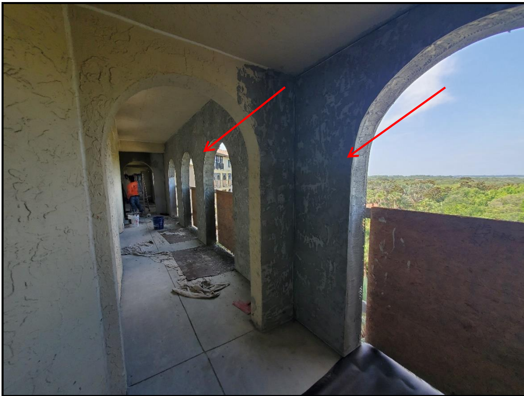
Photograph 13. 6 th floor archway stucco installation in progress.
