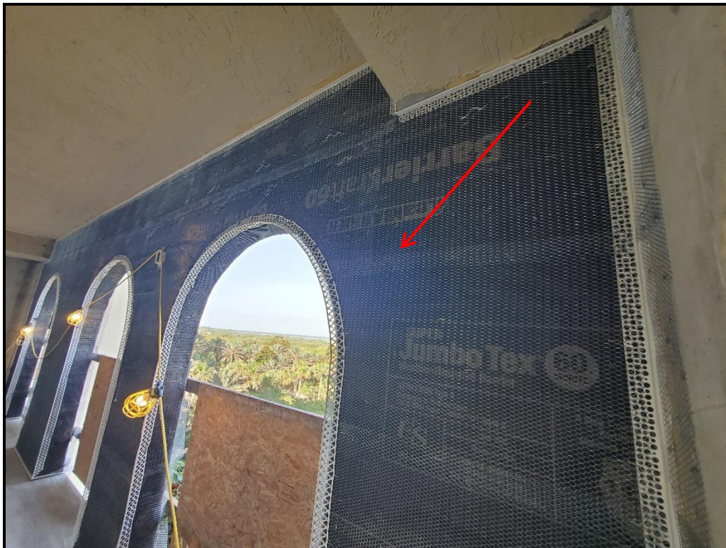
Photograph 1. 6 th floor west walkway stucco accessories and lath installation in progress.
